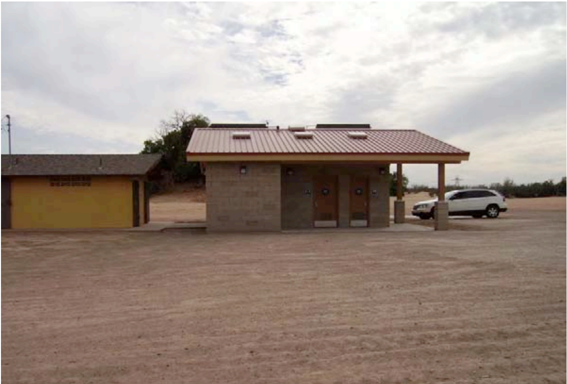
Photograph 4. View of par restrooms to right; closed restroom to left.
