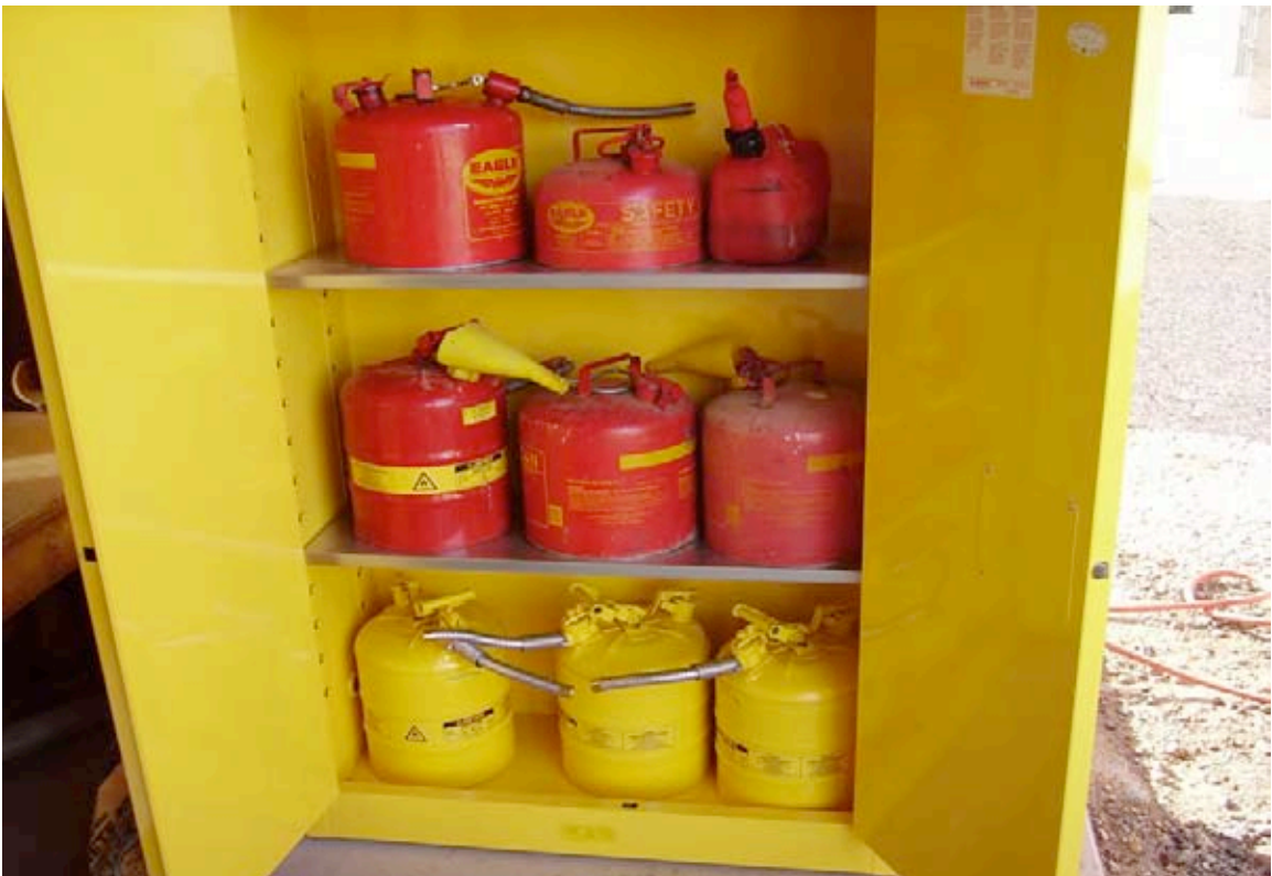
Photograph 8. View of fuel canisters flammable locker at ranger shop area.
