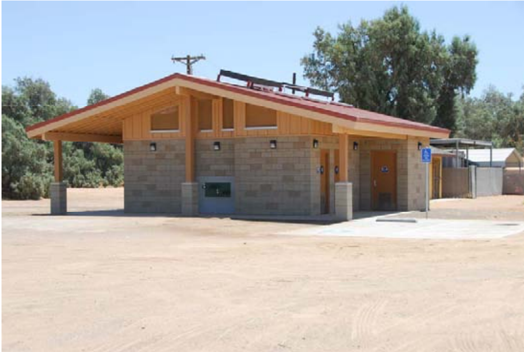
Photo 3.6-2. View of restroom facilities
