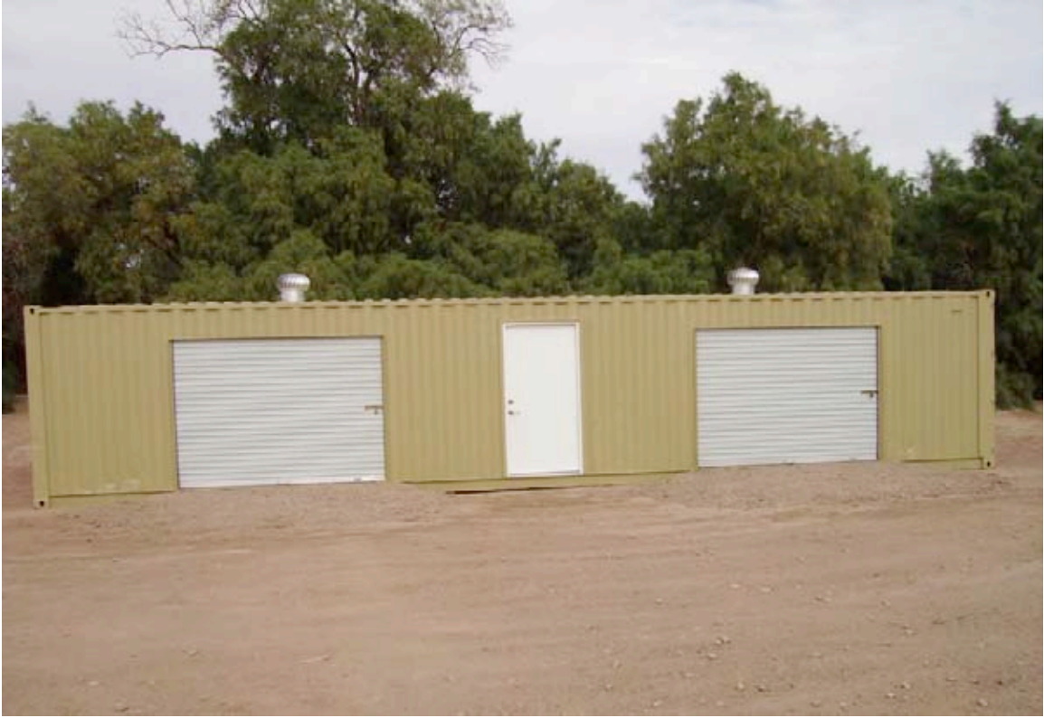
Photograph 5. View of typical park storage building.
