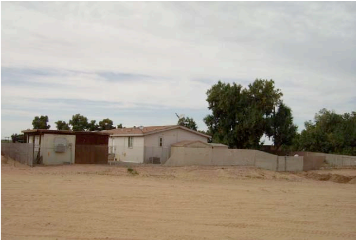
Photograph 6. View of ranger living quarters and shop area to left of residence.
