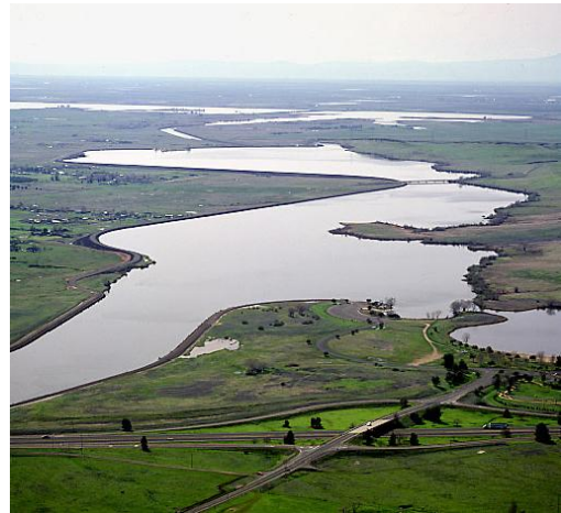
Thermalito Forebay (view southwest)
