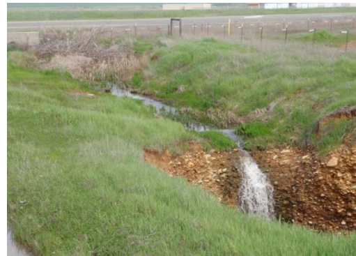
Drainage from north culvert under Larkin Rd.
