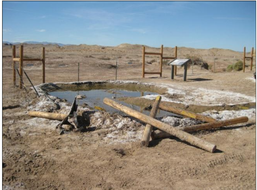
Fences are being repaired.
