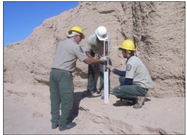
Right: While Ryan holds the new signs on the post, Pete shows Norb Moeller from the Maintenance Department (shadowing our crew for the day), how to properly mount the new signs using our rivet gun.
