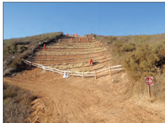
Oakie restoration project #2
