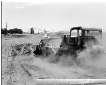
Detail of scrapers
