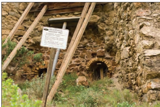
Mine adits, Carnegie SVRA
