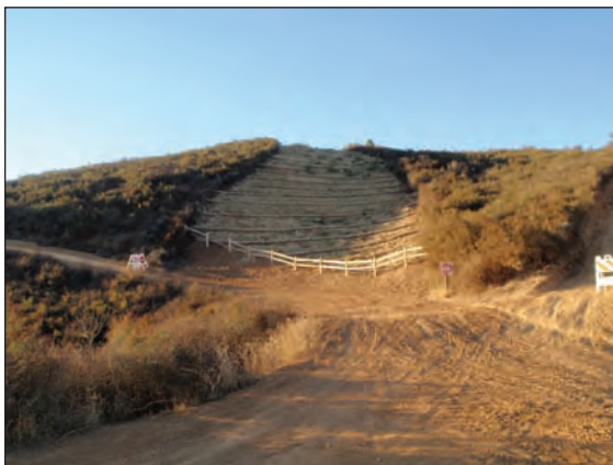
Oakie restoration project #3
