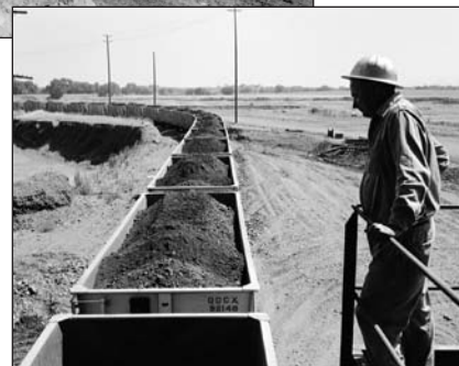
Material on train leaving Clay Pit for dam site
