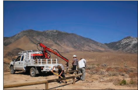
Maintenance on the Trails
