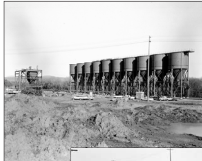
Hoppers used to screen material before transport to dam site
