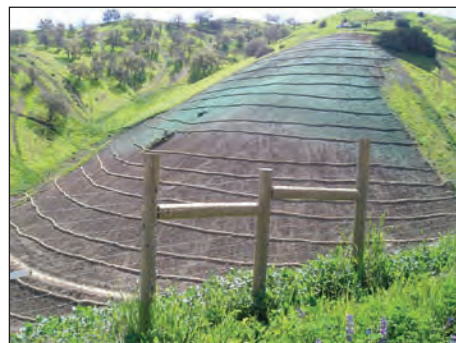
SRI Loop Restoration #4
