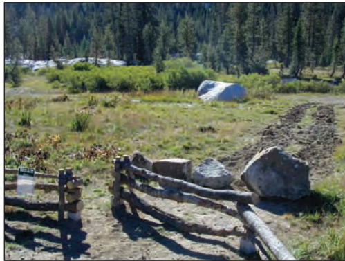
Tahoe National Forest Fence Project
