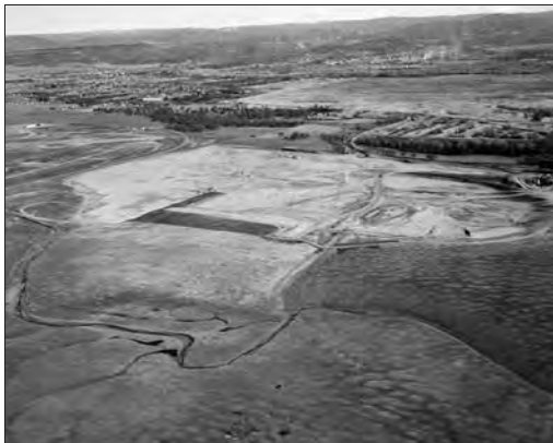
Clay Pit area before soil excavation
