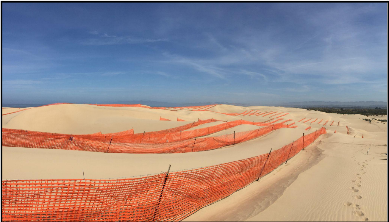
Plastic Fencing Project Installed in Oceano Dunes at the Direction of the SAG. The purpose of the fencing is to halt sand saltation in the dunes (photo: Will Harris).
