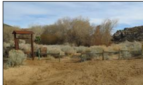
New fence installed at Butterbredt Spring
