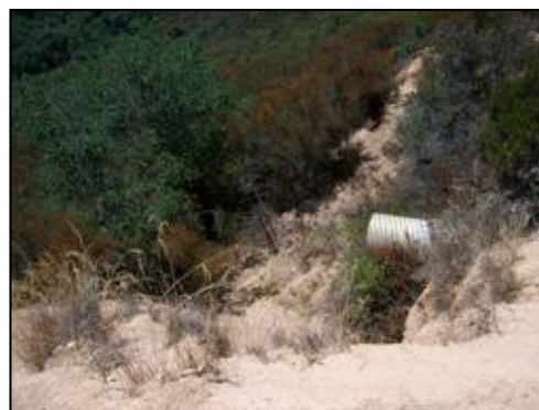
Olive Orchard culvert
