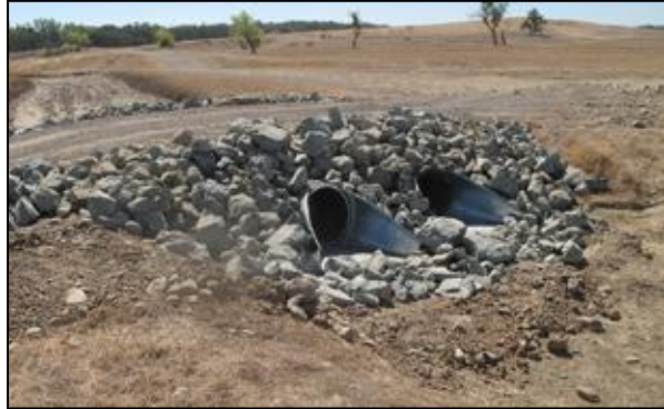
New culvert installation at Clay Pit SVRA
