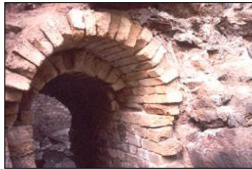
Lime Kiln Tunnel at Carnegie SVRA
