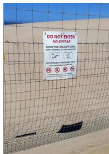
Six-foot “no-climb” fence
