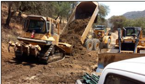
Equipment operators moving sediment to project site
