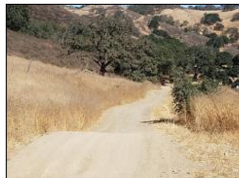
Rancho Road one year after rehabilitation
