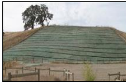
Restoration Project - During
