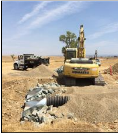
Heavy equipment operators installing the culvert
