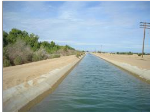
South Alamo Canal
