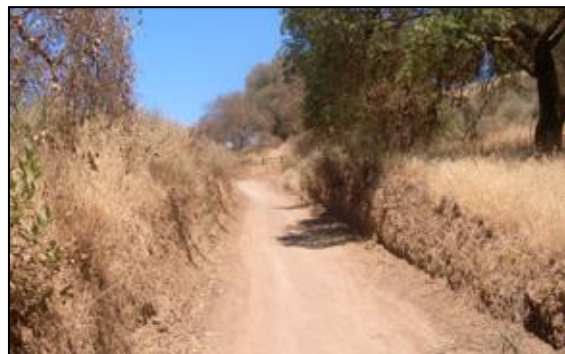
Rancho Road before rehabilitation
