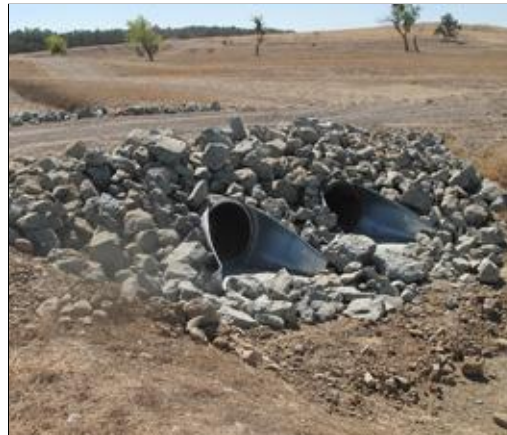
Culvert in the Drainage Management Area
