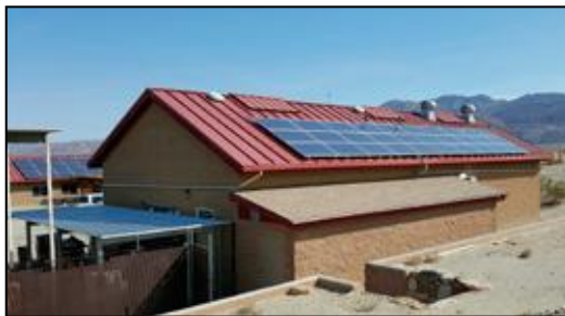
Roof installation of solar panel system
