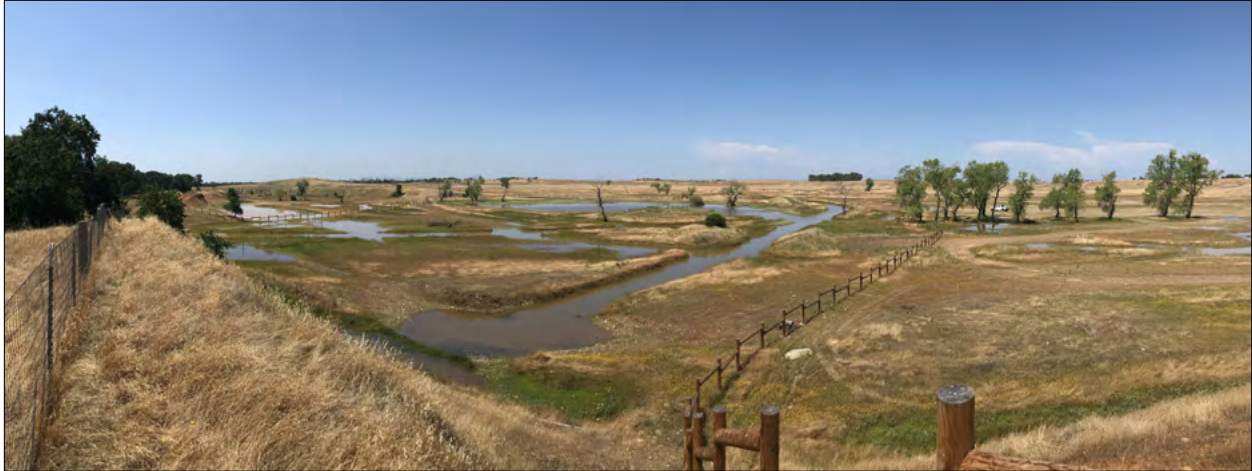
Figure 85. Clay Pit SVRA Drainage Management Area Restoration Project.
