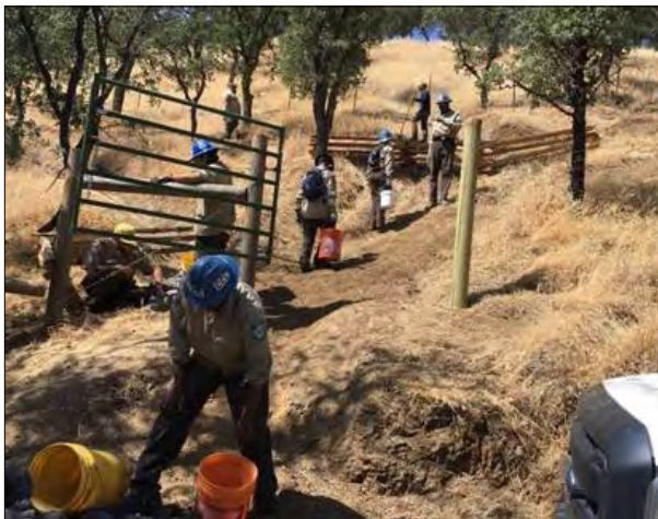
Figure 83. On the Black Bear RMA Project, the CCC crew placed a rock on the trail's edge to prevent erosion.
