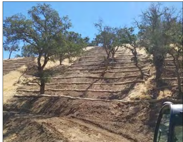
Figure 84. Black Bear Resource Management Area Restoration Project—straw waddle placement.
