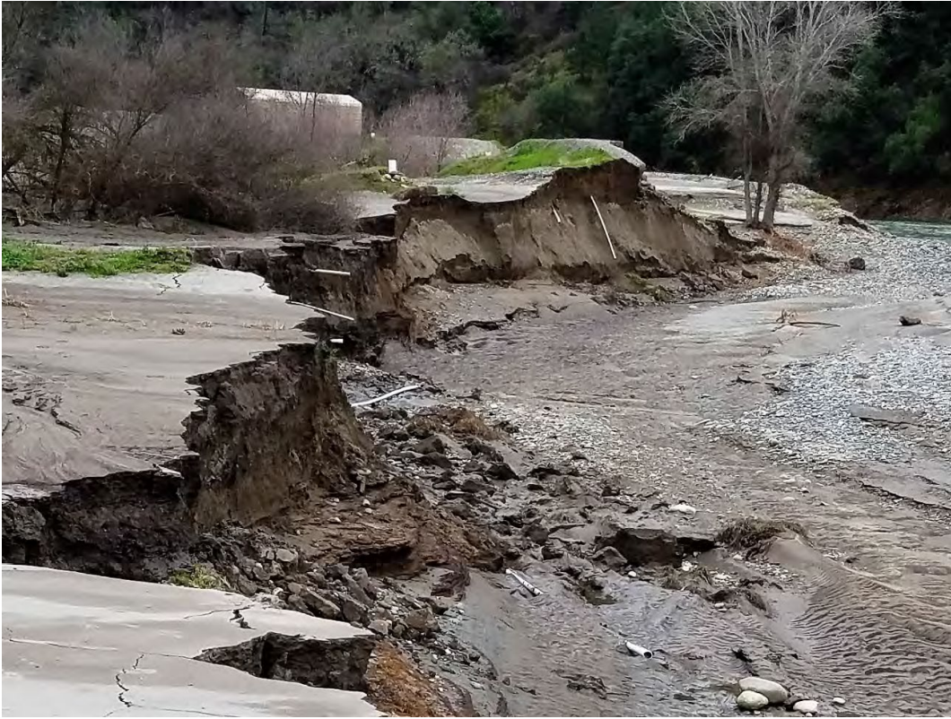
Bank on west side of MX Track eroded by February 2017 high water flow along channel braid.
