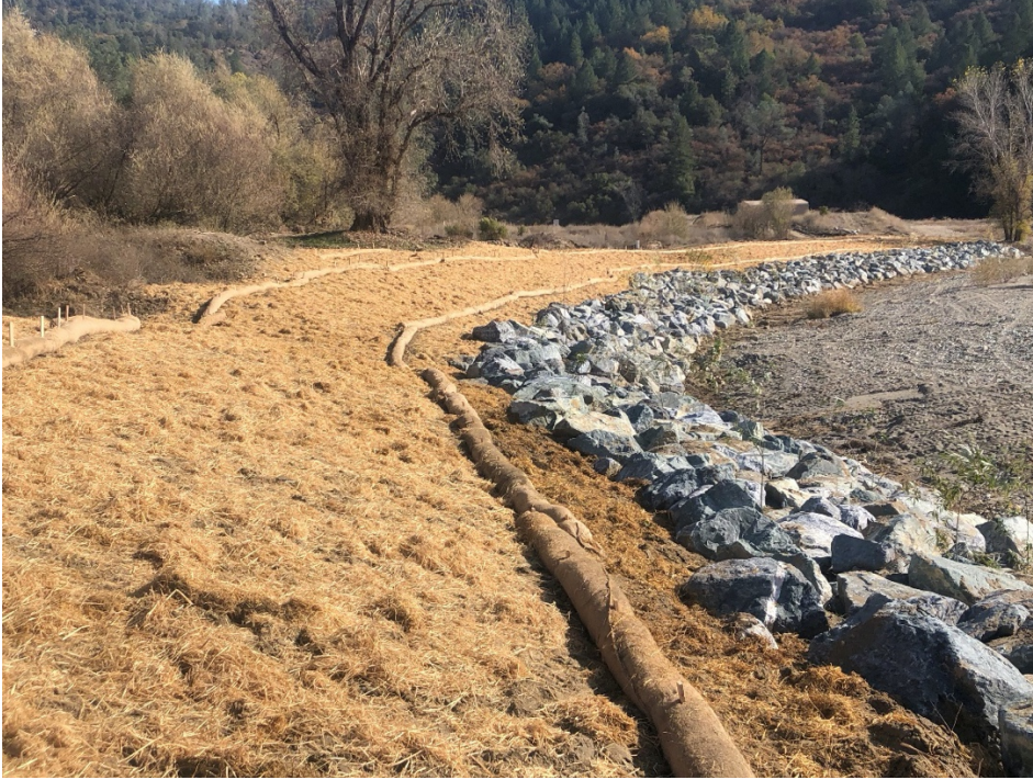
Completed Cut Bank Mitigation Project, November 2019.
