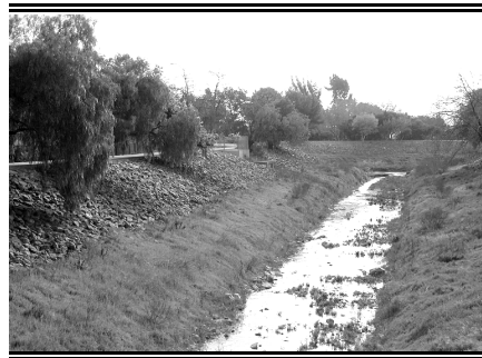
Dry Creek channel with pedestrian path beyond
