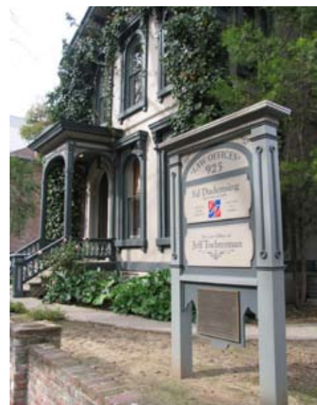
The former Van Voorhies Mansion, built in the Italianate architectural style, has undergone historic restoration and is now used as offices.
