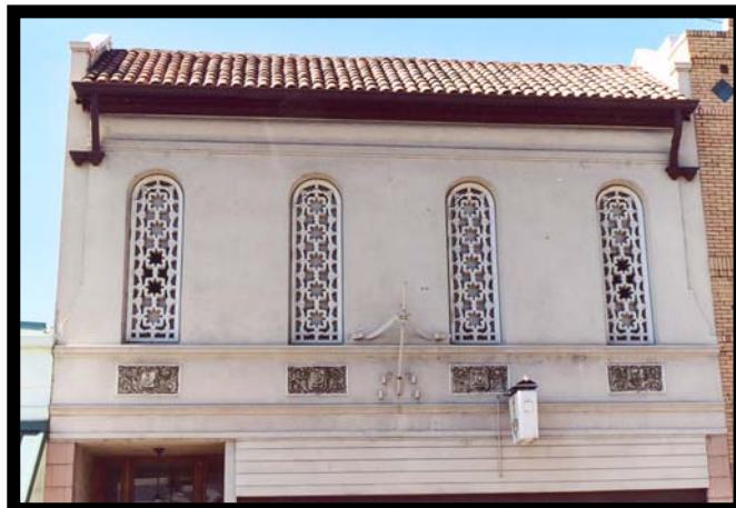
Figure 38: Masonic Hall, Spanish Eclectic, Built 1858, Remodeled 1929, 16 South Washington Street
