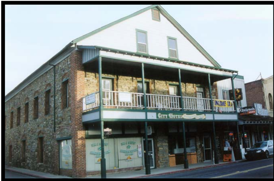
Figure 31: City Hotel, Constructed 1853, 139-145 South Washington Street, One of Sonora’s first substantially stone buildings
