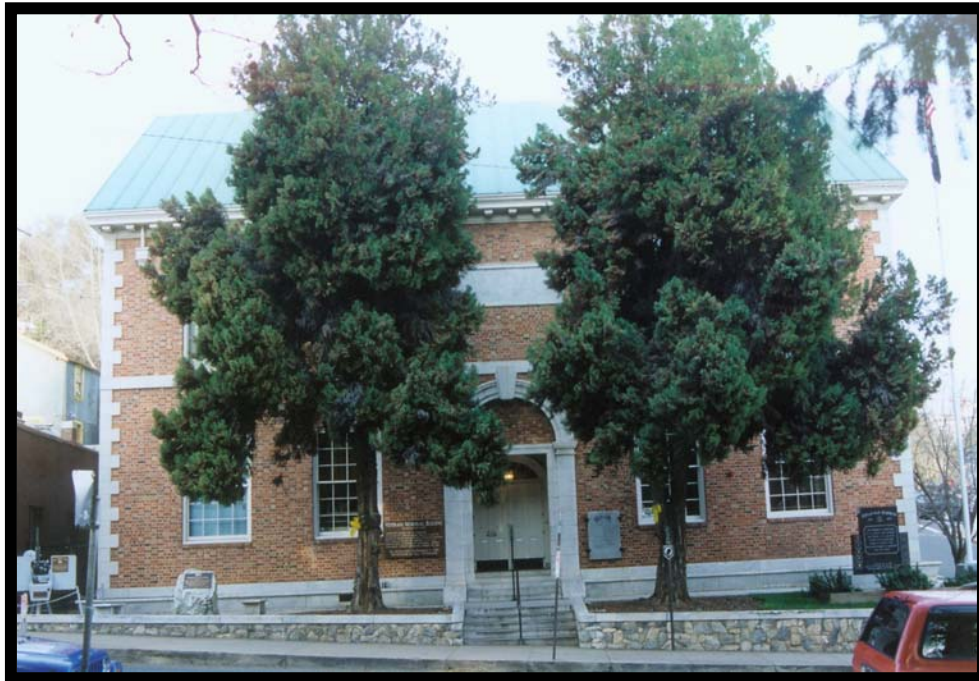
Figure 40: Veterans Memorial Hall, Constructed 1933, 9 North Washington Street, An example of Sonora's Colonial Revival Architecture
