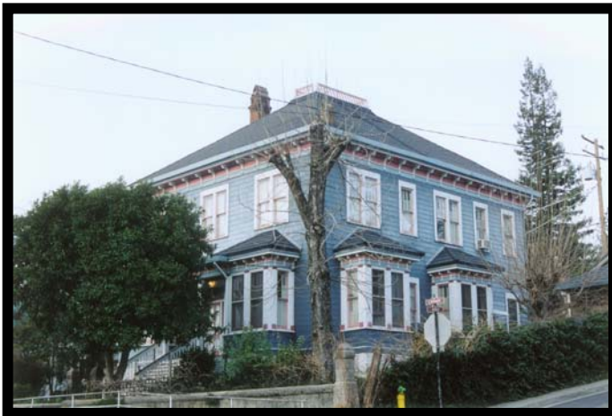
Figure 24: Nicol Mansion Constructed 1887, 313 South Stewart Street
