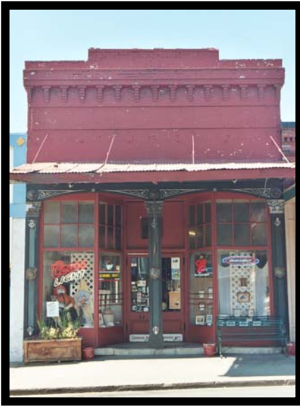
Figure 32: Servente's Constructed 1856, 64 S. Washington, The only remaining building in Tuolumne County with an iron storefront ( by Sutler Iron Works). Formerly Charles Freidenberg Dry Goods; Haag's Cigars & Groceries; Presently Servente's Groceries & Liquors.
