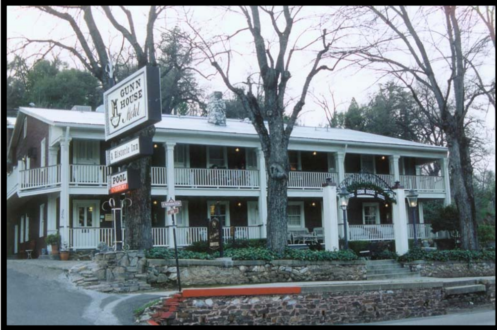
Figure 29: Gunn House, Constructed 1852, 186 South Washington Street, A Sonora adobe – Believed to be the oldest building in Sonora, Served as the county hospital in 1852 and later as Bisordi's Rosa Italia Hotel
