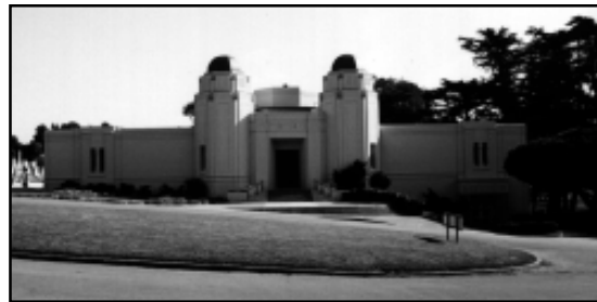
C. Hills of Eternity 1301 El Camino Real Rating: Historic Resource
