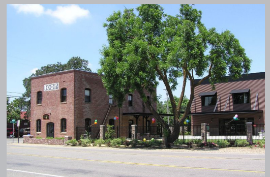
Adaptive reuse of former Odd Fellows Hall in Clements into a facility for manufacture and retail of chocolate products involved a related new construction component 20% Historic Tax Credit Project
