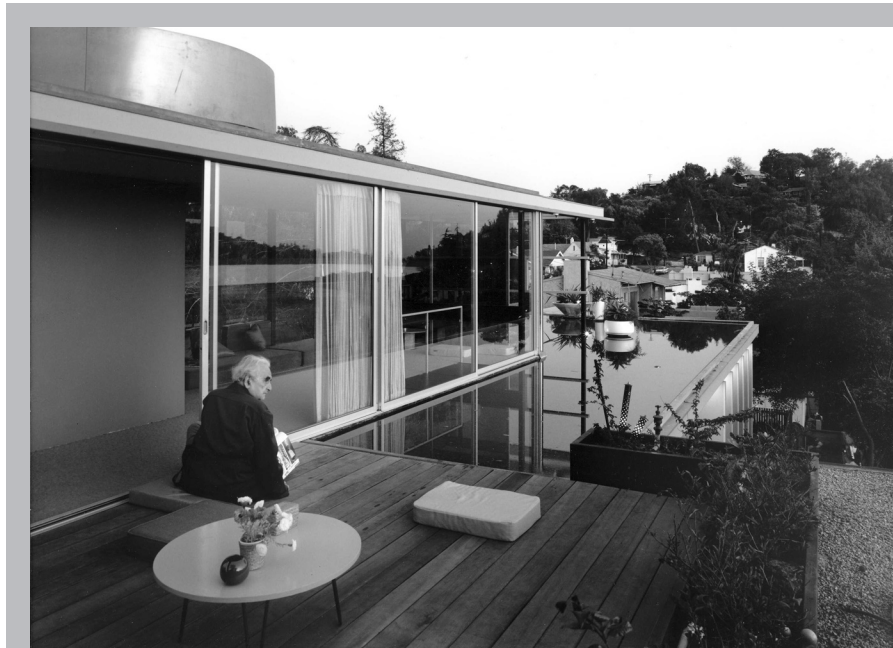
In 1932, Richard Neutra designed the Silver lake Research House as his family residence. Recognized as one of the earliest “modern” houses in the US and an outstanding example of the International Style, it burned in 1963. Four years later, Richard Neutra and his son, Dion, collaborated in designing a new house on the original foundation. Reflecting Neutra’s changing aesthetic through a visual network of reflective and transparent planes which integrates interior and exterior space, the Neutra VDL Research House II is a Los Angeles Cultural Monument and was listed by World Monuments Watch as one of the 100 Most Endangered World Monuments in 2000.
