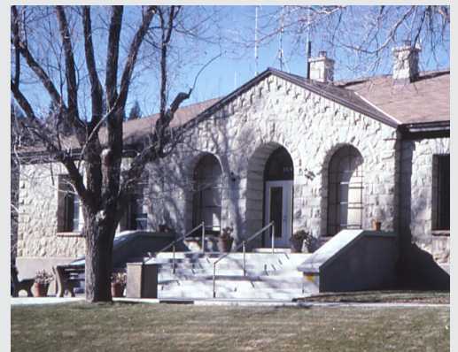
Alpine County Courthouse, Markleeville. Built in 1916 on plans by Reno, Nevada architect, Frederick DeLongchamps. It was the first building to be listed in the National Register in tiny Alpine County (pop. 1200).
