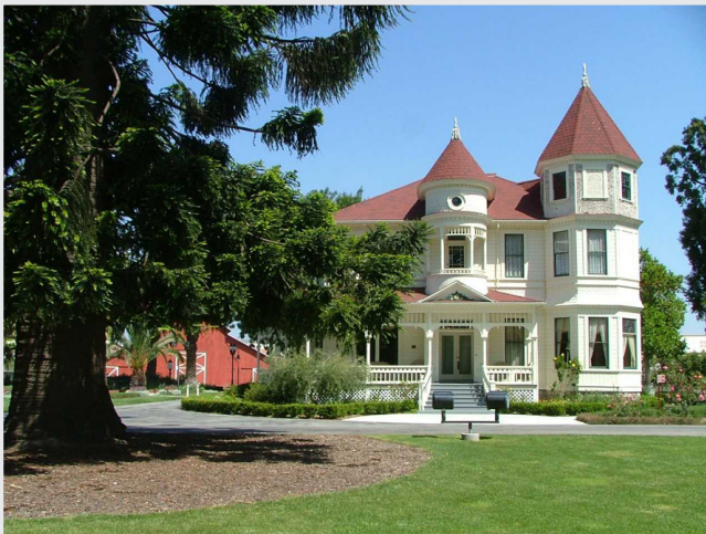
Once part of the 10,000-acre Camarillo Ranch in Ventura County, this 1892 Queen Anne, owned by the City of Camarillo, is listed as a California Point of Historical Interest and on the National Register.
