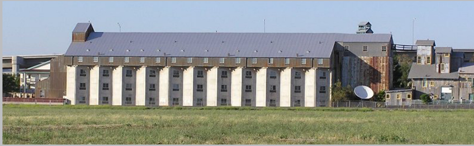
Irvine Bean and Grain Growers Building, Irvine Adaptive reuse of lima bean and grain silos and warehouse space into hotel – 20% Historic Tax Credit Project
