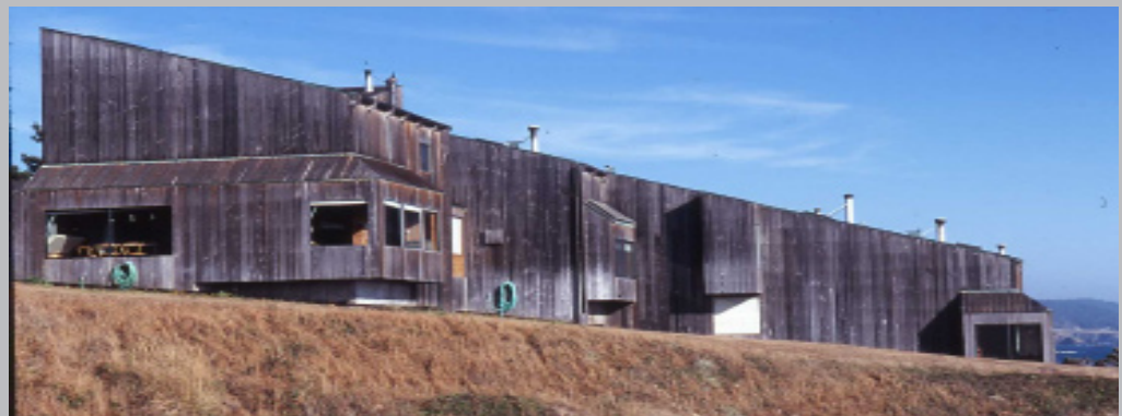
The Sea Ranch, Condominium 1, Sonoma County is an exceptional example of 1960s Modernism. Designed by Charles W. Moore, Donlyn Lyndon, William Turnbull, Jr., and Richard Whitaker (MLTW) in 1965 as an environmentally sensitive second-home development, each 24-foot redwood cube features glass bays with window seats, solariums, terraces, decks, and walled gardens with ocean views.
