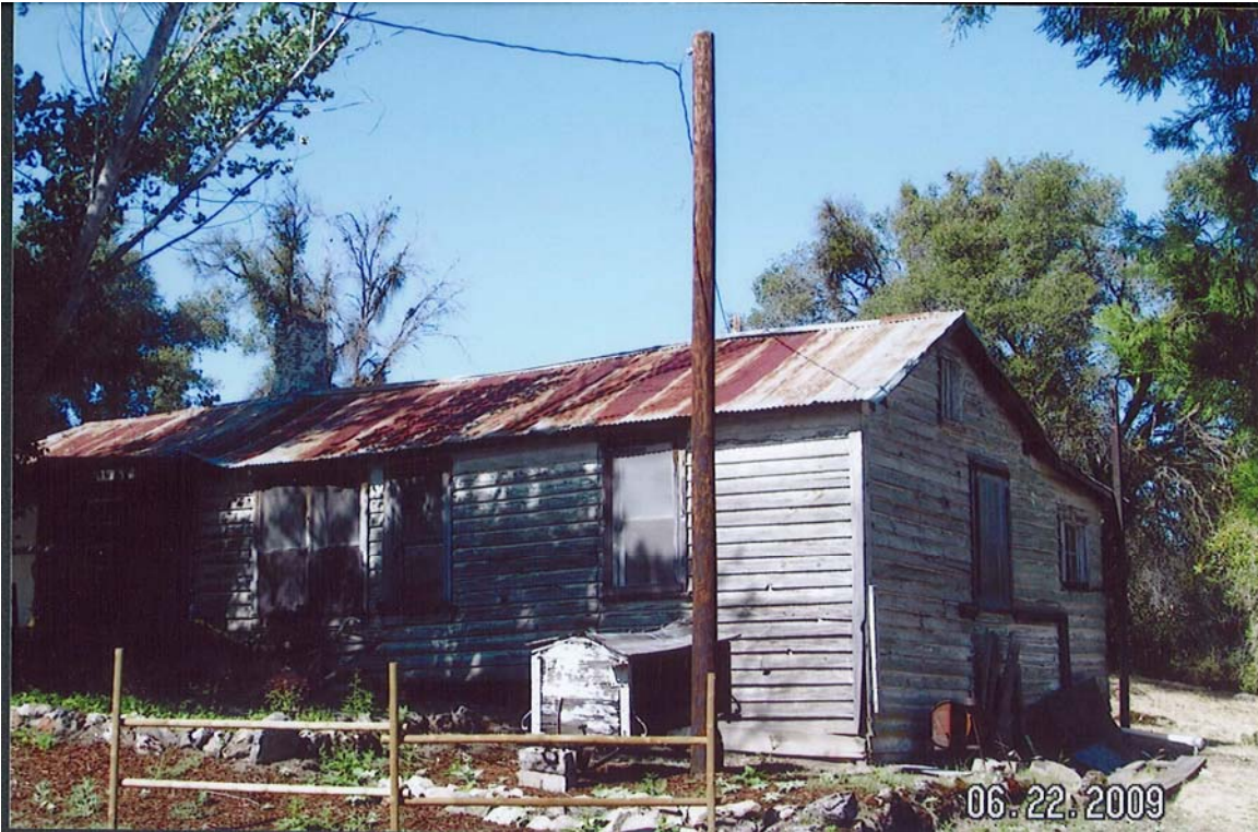
#5 Northeast corner of wooden portion
