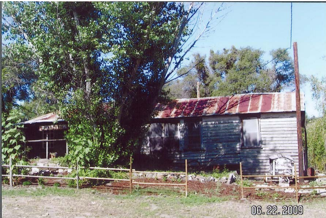
#4 East side of entire building
