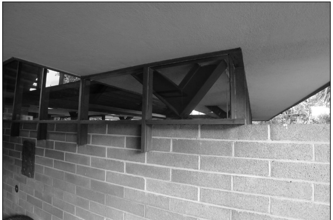
Illustration 5. Glass corner at Living Room reveals steel structural supports for roof.
