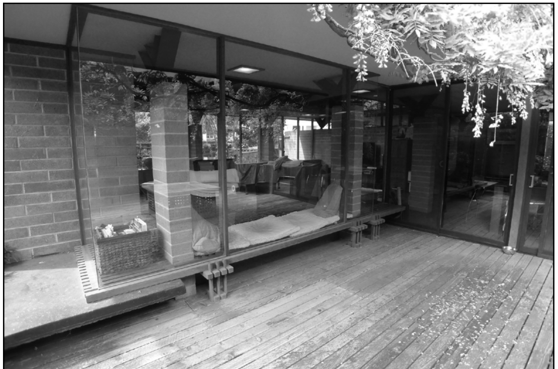
Illustration 7 ( below ). Living Room seen from courtyard patio.
