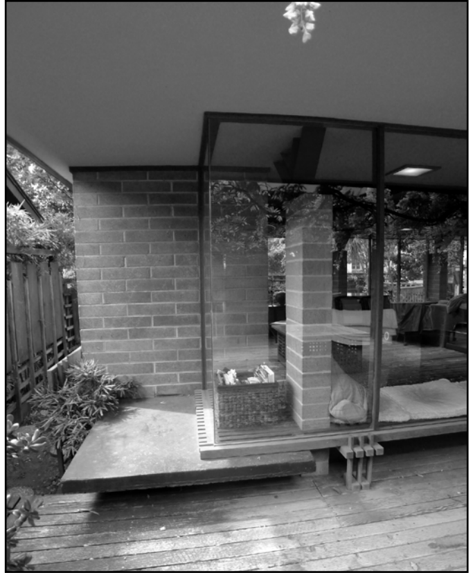
Illustration 6 ( right ). Living Room corner seen from courtyard patio showing floating hearth extension, slatted bench, and butt joint at glass corner.
