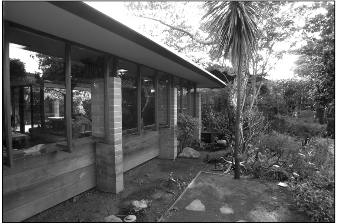
Illustration 4. Living Room exterior showing horizontal "shelf" at glass curtain walls between masonry piers and wide roof overhang.
