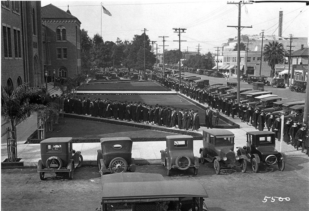
View from the Gwynn Wilson Student Union building, looking north at Bovard and University Avenue (now Trousdale Parkway). Photograph 1925, Los Angeles Public Library.
