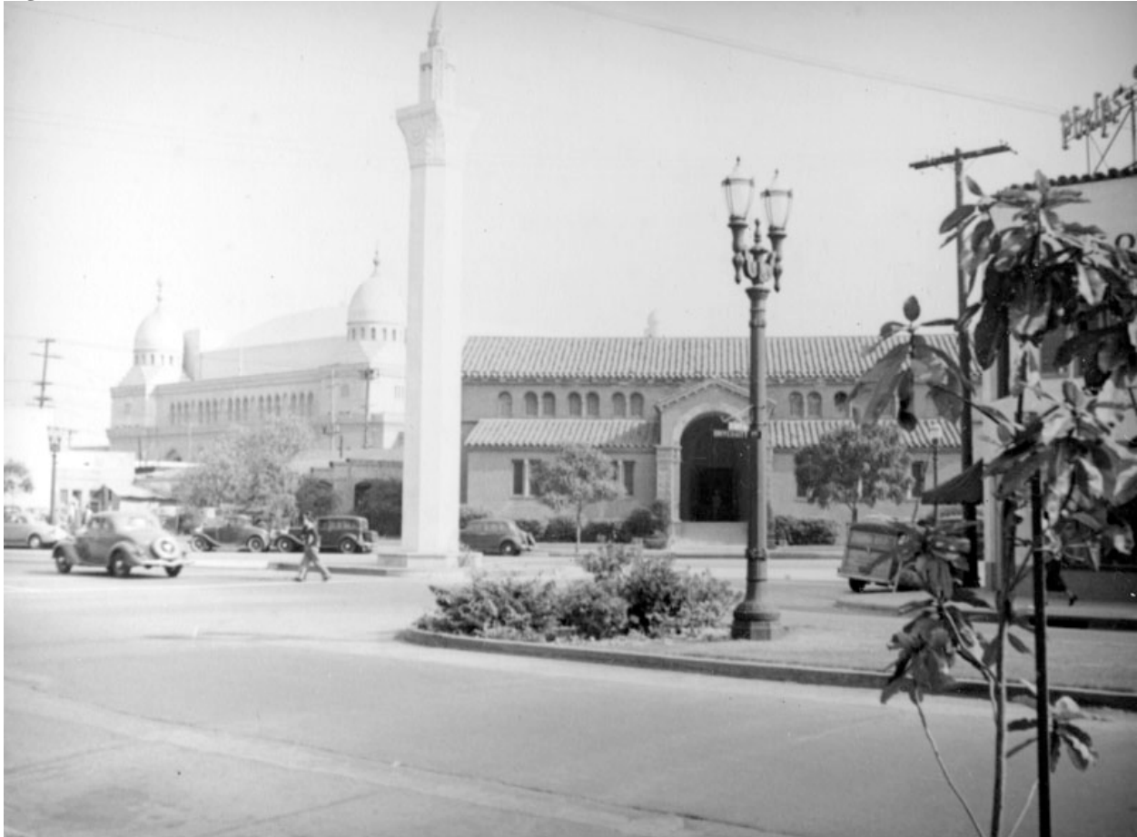
USC Entrance at Jefferson, Hoover, and University Avenues. Buildings from left to right include the Shrine Auditorium, the original University Branch Library (demolished) and Phelps-Terkel Men's store. Photograph 1937, Los Angeles Public Library.
