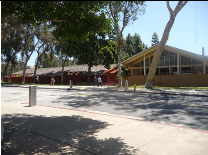
Plate 1. Primary (West) Elevation, View to East (PCR 2011)
