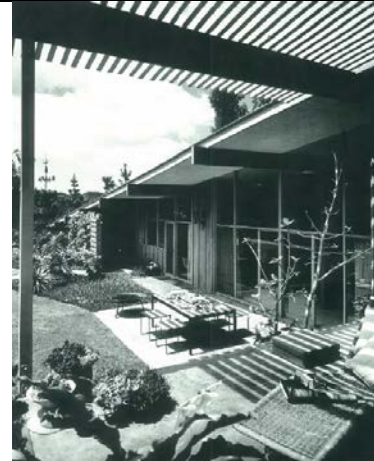
Plate 40. Edward Fickett designed Home, 1955 (LA Conservancy)
