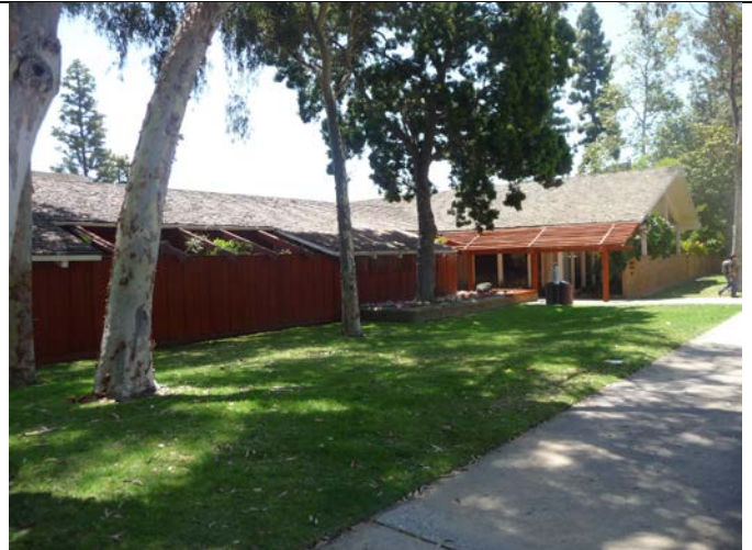
Plate 2. Primary (West) Elevation, View to Southeast (PCR 2011)
