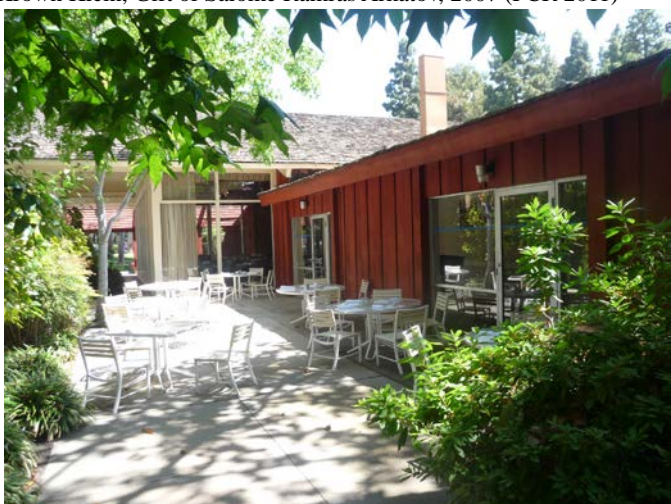
Plate 29. Outside Patio, Accessed from South Hallway, View to North (PCR 2011)
