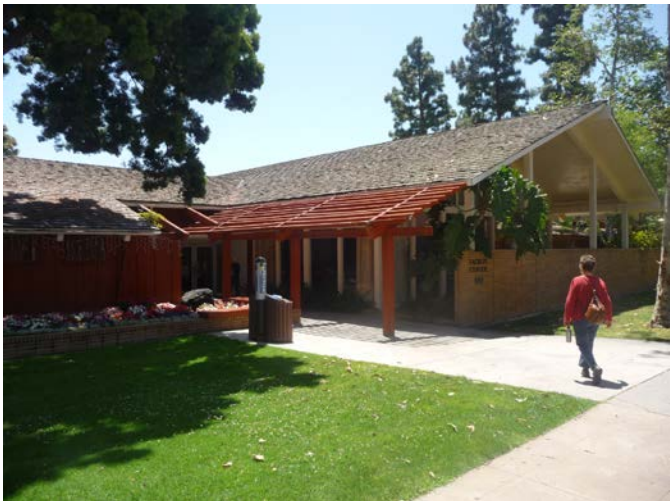
Plate 3. Primary (West) Elevation, View to Southeast (PCR 2011)
