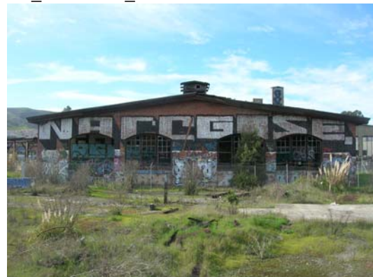
CA_SanMateo_SPRoundhouse6. The east facade Southern Pacific Roundhouse, camera looking west
