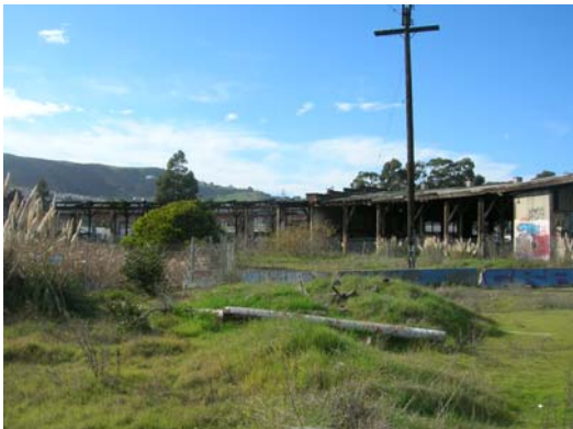
CA_SanMateo_SPRoundhouse5. The south facade of Southern Pacific Roundhouse, camera looking west.
