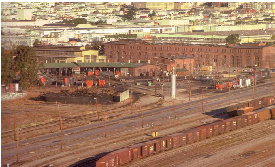
Historic Illustration 6. Roundhouse and turntable with other yard buildings (no longer extant) in 1975. Source: Anthony J. Thompson and John R. Signor ( Southern Pacific's Coast Line Pictorial , Wilton, CA: Signature Press, 2000), 39.
