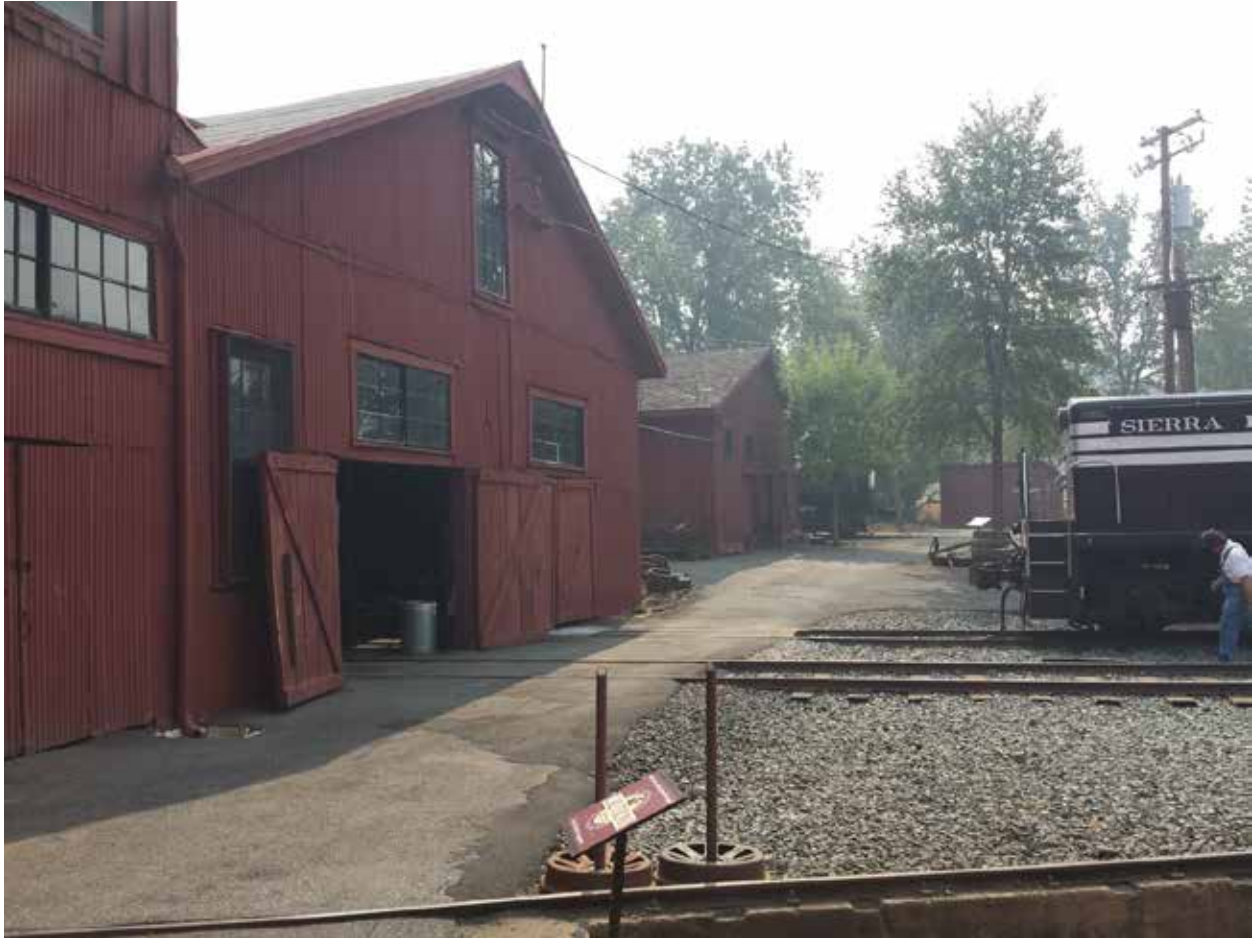
3. Machine shop exterior
