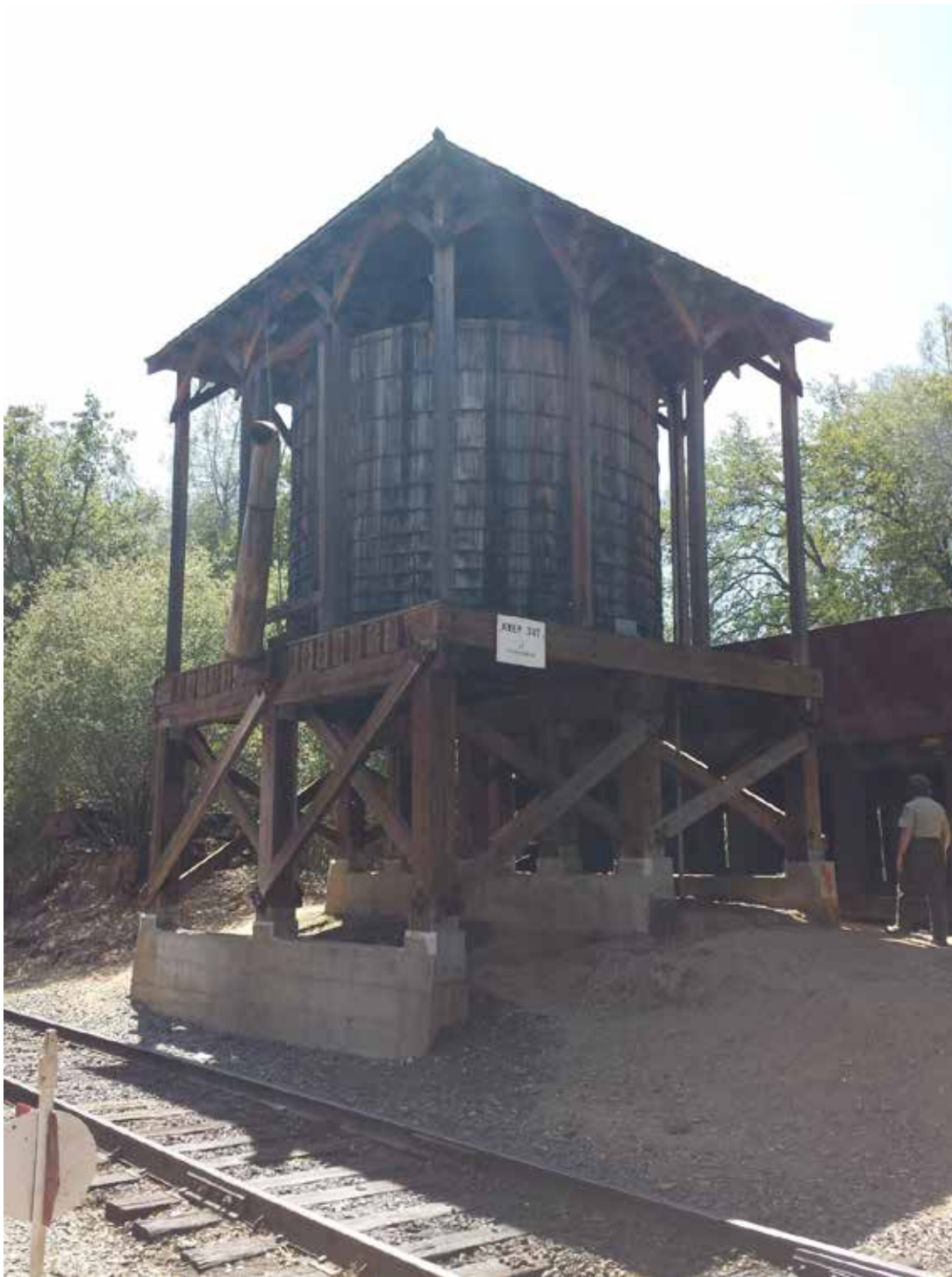
7. Sierra water tank (reconstructed)
