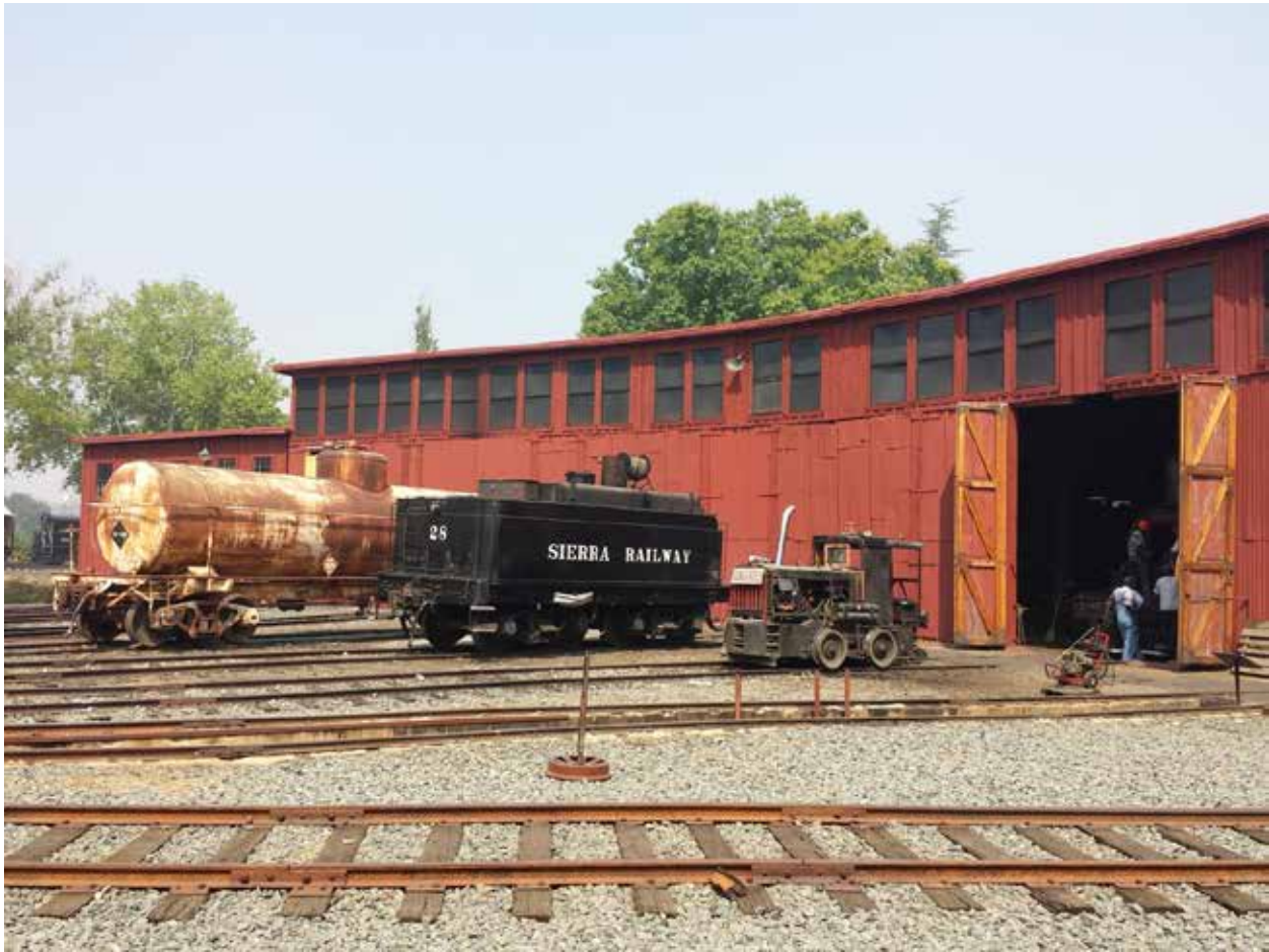
2. Exterior view of roundhouse.
