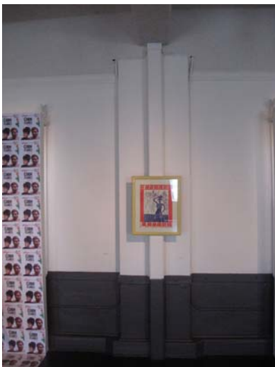
Detail of concrete column in multi-purpose room. (Edgar Garcia)
