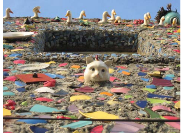
South façade. Detail of embedded and projecting ceramic pieces. (Edgar Garcia)
