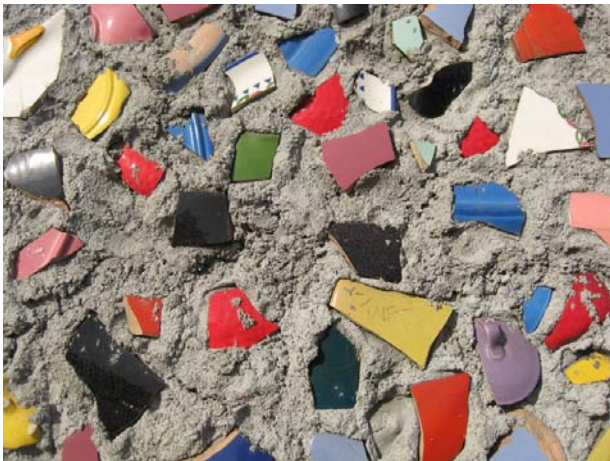
South façade. Detail of embedded ceramic pieces. (Edgar Garcia)
