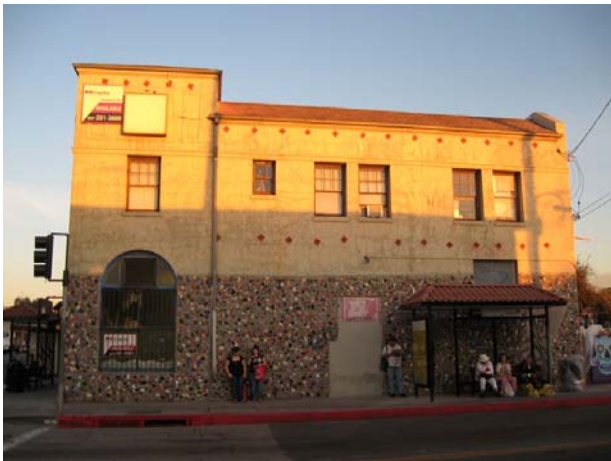
West façade. (Edgar Garcia)
