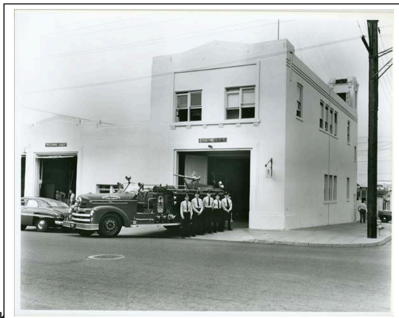
(Image 14: Taken from the street, showing the relocation of the radio antenna. There is also an unobstructed view of the north facade.)
