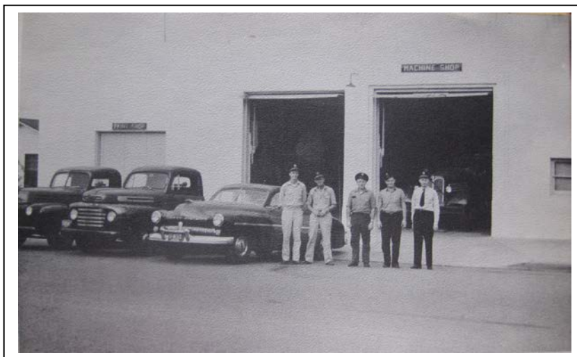
(Image 13: This photo, estimated in 1951, (the Mercury is a '49 or '50) shows the southern addition moved forward flush with the rest of the building and labeled "Paint Shop", with two garage doors instead of one as well as a smaller northern window to accommodate an office.)
