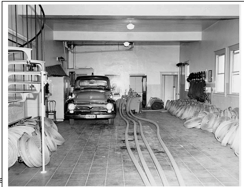
(Image 19: This image, taken from the front part of the repair portion of the machine of the front part of the bning system used in the ceiling to reduce beams, providing a more open floor space.)
