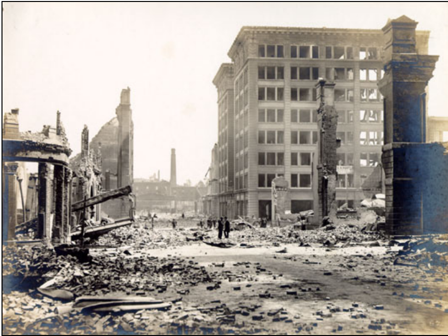
Rialto Building after the 1906 Earthquake and Fire. Photograph Courtesy of the San Francisco Public Library Historical Photograph Collection.
