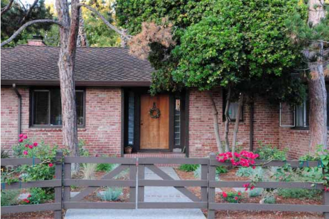
120 Arroyo Way, Front Door, Approximately Viewing North-East
