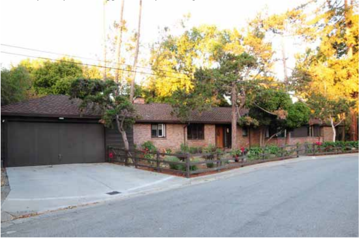
120 Arroyo Way, Front, Approximately Viewing East
