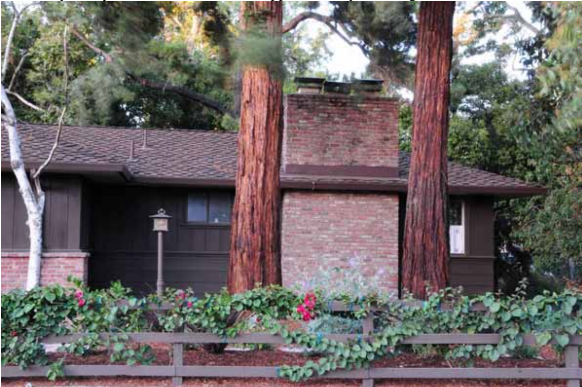
120 Arroyo Way, 1949-1950 Addition, Approximately Viewing North-East
