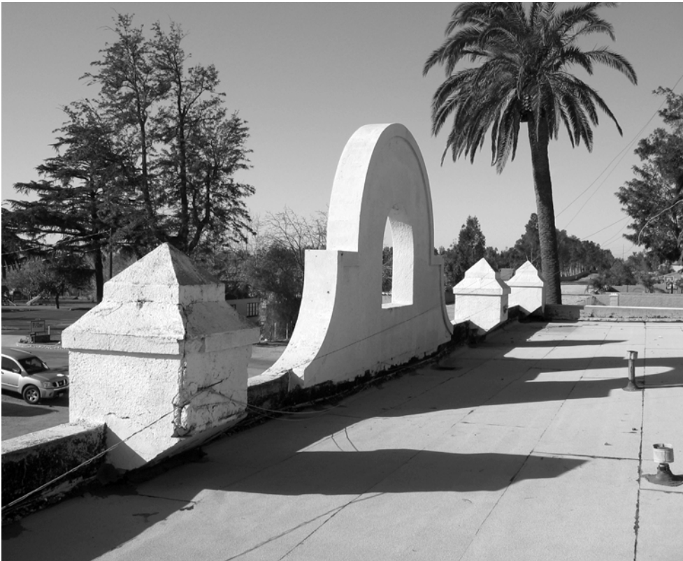
Figure 20 View of decorative arch and typical pilaster caps from roof.
