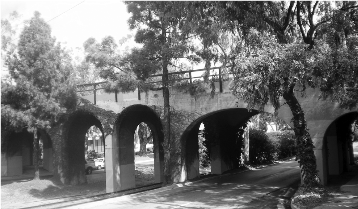
Figure 16 Pacific Electric Railroad Bridge, erected 1913, Irving Gill Architect, Torrance, CA.
