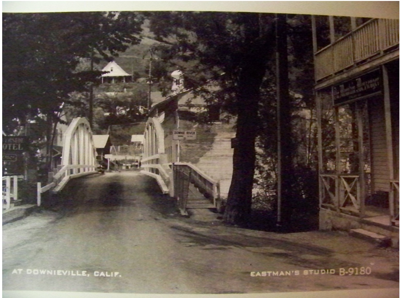
Figure 4. Historic photo of Jersey Bridge, date unknown
