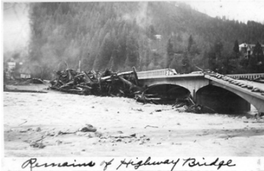
Figure 2. Historic photo of damaged highway bridge, 1937
