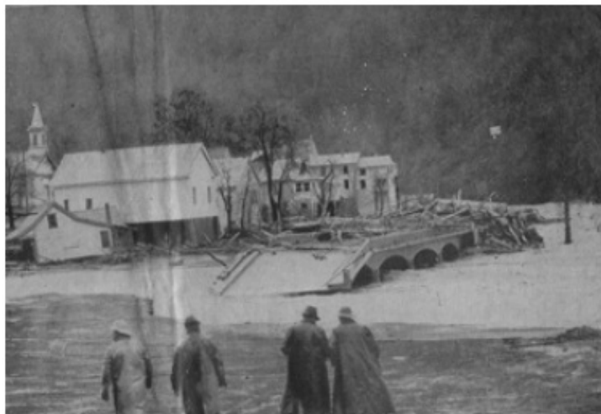
Figure 3. Historic photo of damaged highway bridge, 1937
