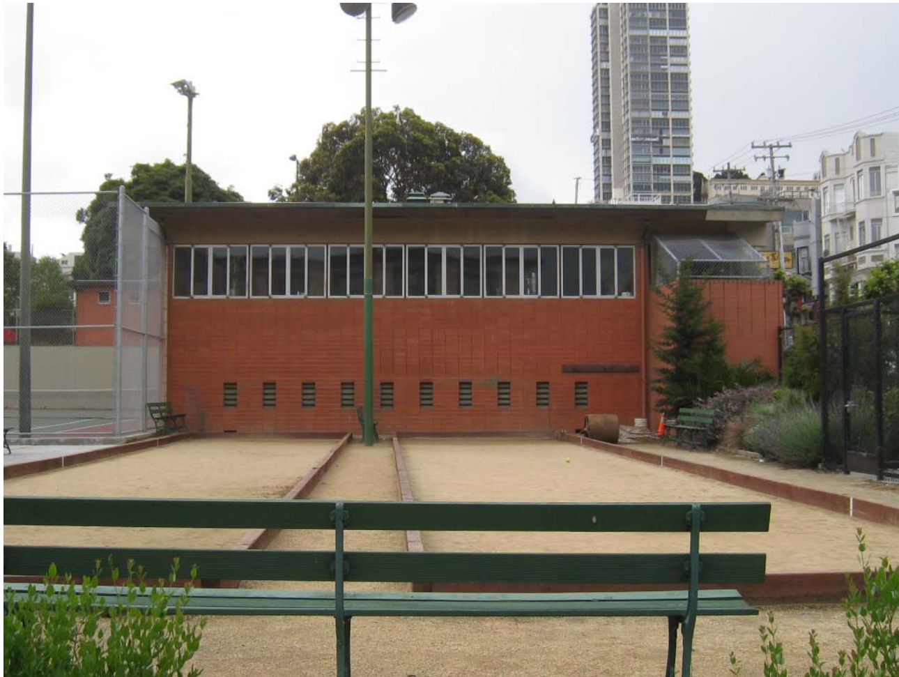
North Beach Branch Library, San Francisco. View of North Elevation. Taken 27 April 2010 by Johanna Street.
