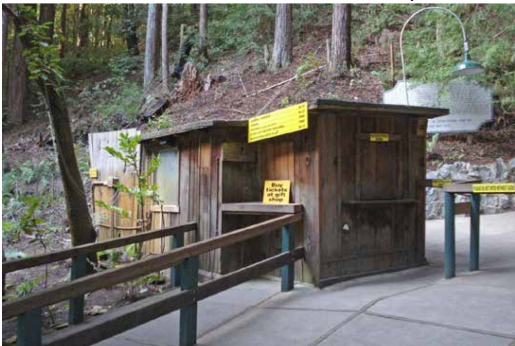
Photo #11 – Exterior of 1941 Ticket Booth north end, taken January 22, 2013
