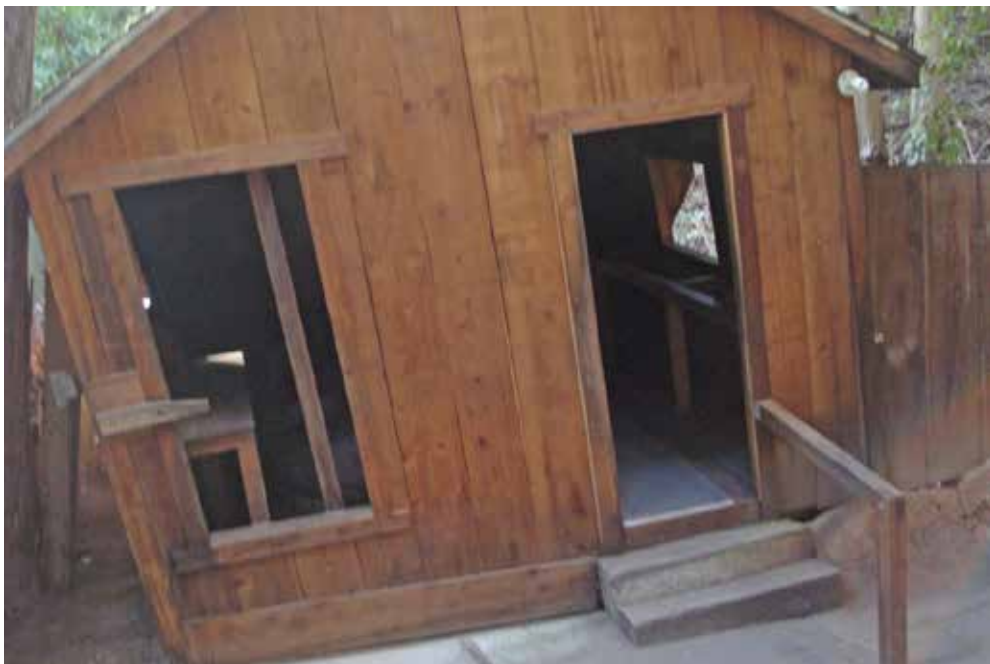
Photo #3 - North end of shack – same perspective as 1941 photo
