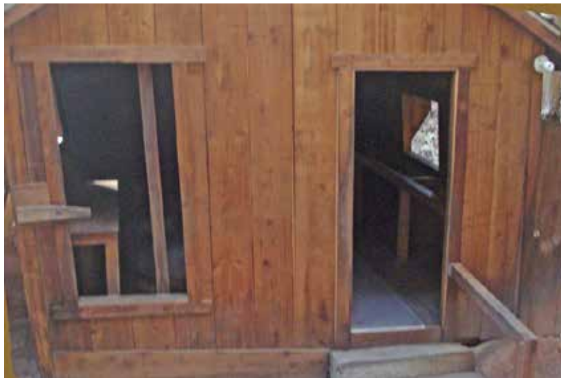
Photo #7 - North end of shack – same perspective taken January 15, 2013
