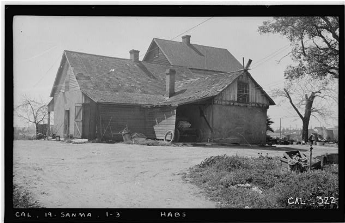
Figure No. 3. Historic American Buildings Survey Photographed by Henry F. Withey, April 1936. VIEW FROM NORTH-EAST, REAR. Call no.: HABS CAL, 19-SANMA, 1-3, CAL-322
