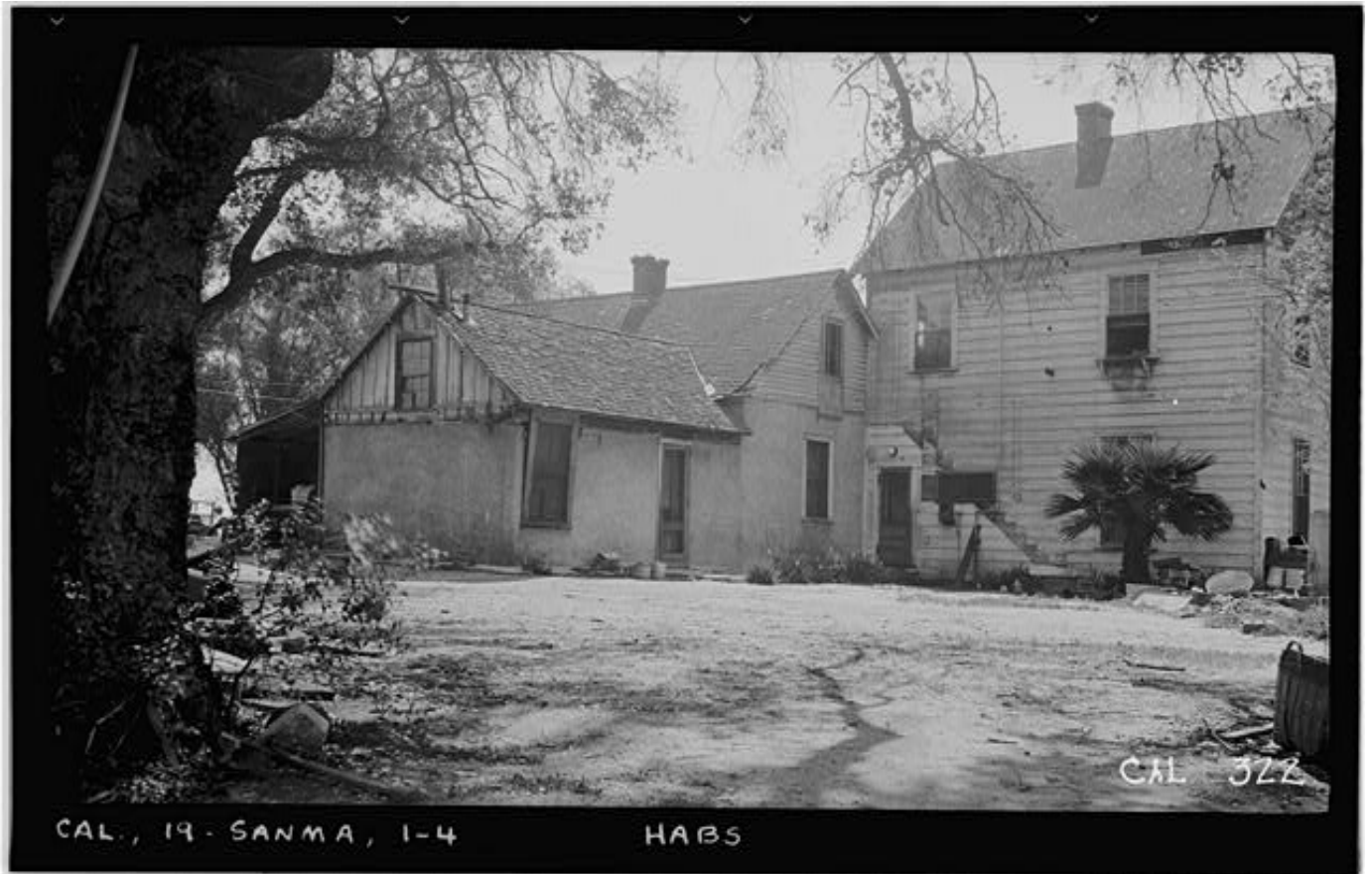
Figure No. 4. Historic American Buildings Survey Photographed by Henry F. Withey, April 1936. VIEW FROM NORTH-WEST, REAR. Call no.: HABS CAL, 19-SANMA, 1-4, CAL-322
