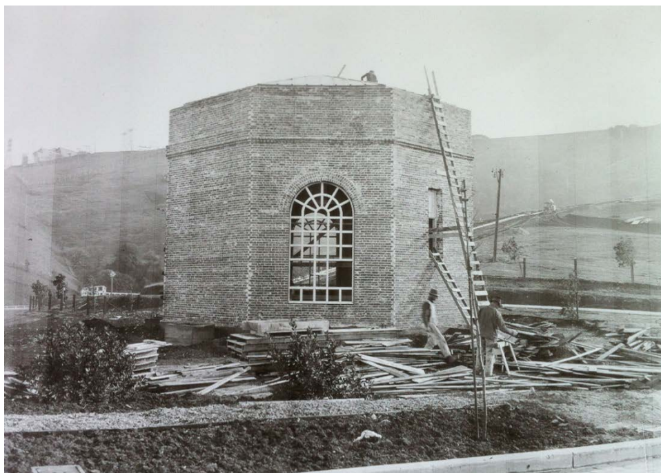
Figure 3: Memorial Hall under construction, looking south, circa 1924. Photo from the collection of the Crockett Museum and Historical Society.
