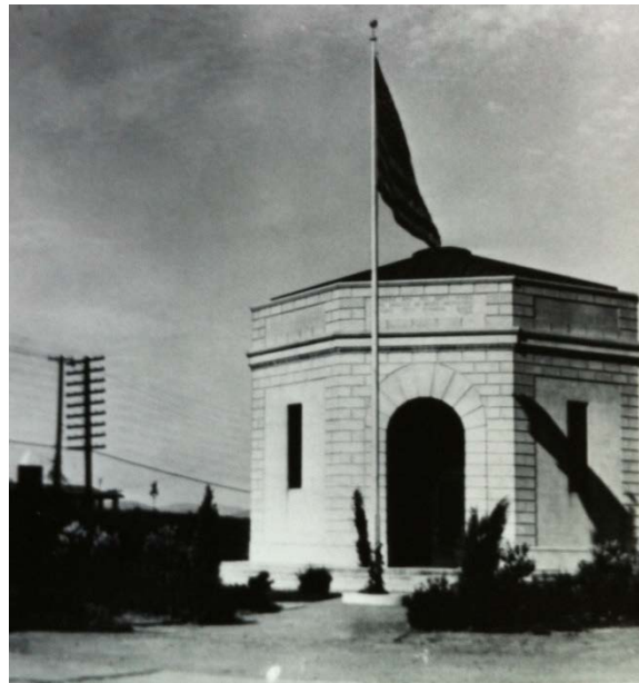
Figure 8: Memorial Hall after completion with landscaping, circa late 1920s. Photo from the collection of the Crockett Museum and Historical Society.
