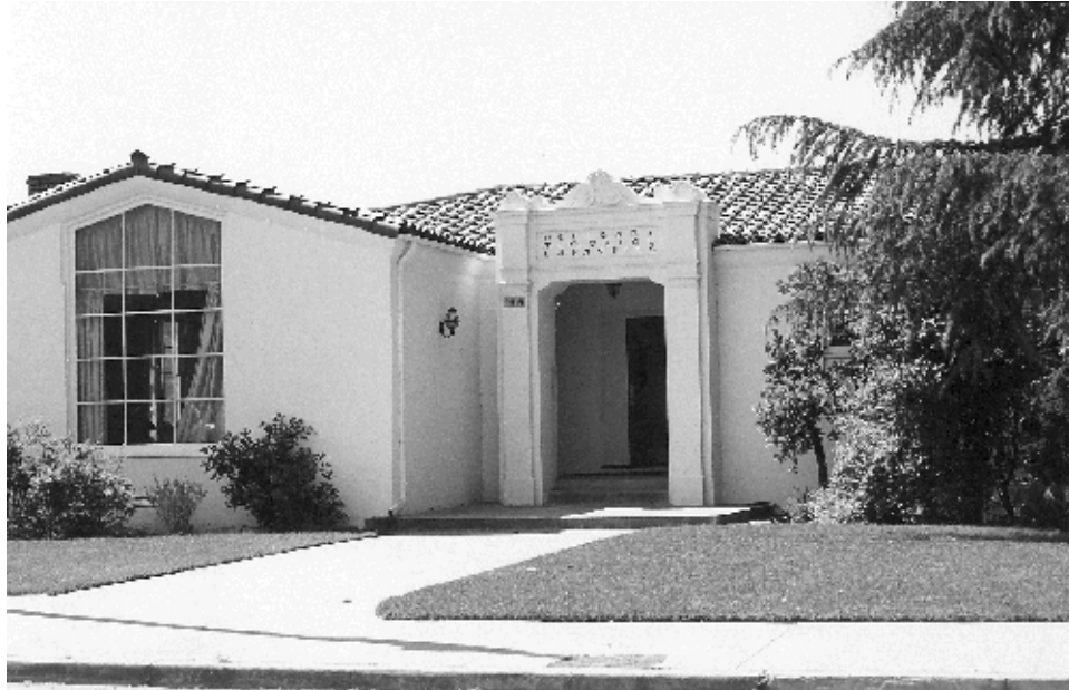
Figure 11: Lafayette Veterans Memorial Building 1939. Image from http://www.lafayetteveterans.org/history.html
