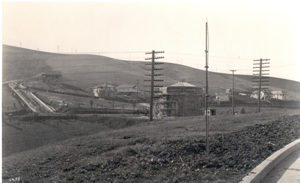
Figure 5: Memorial Hall under construction, looking southwest, circa 1924. Photo from the collection of the Crockett Museum and Historical Society.
