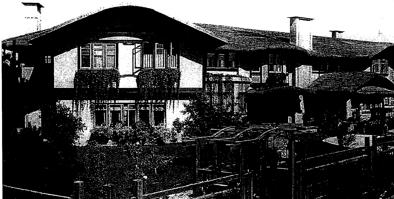
Freeman House exterior detail, c. 1915. Source: Heineman Papers, Greene and Greene Archive.
