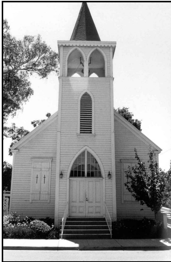
St. Raymond's Church, Alameda County, California. Listed in the National Register of Historic Places on April 12, 2006, at the local level of significance for its architectural qualities.
