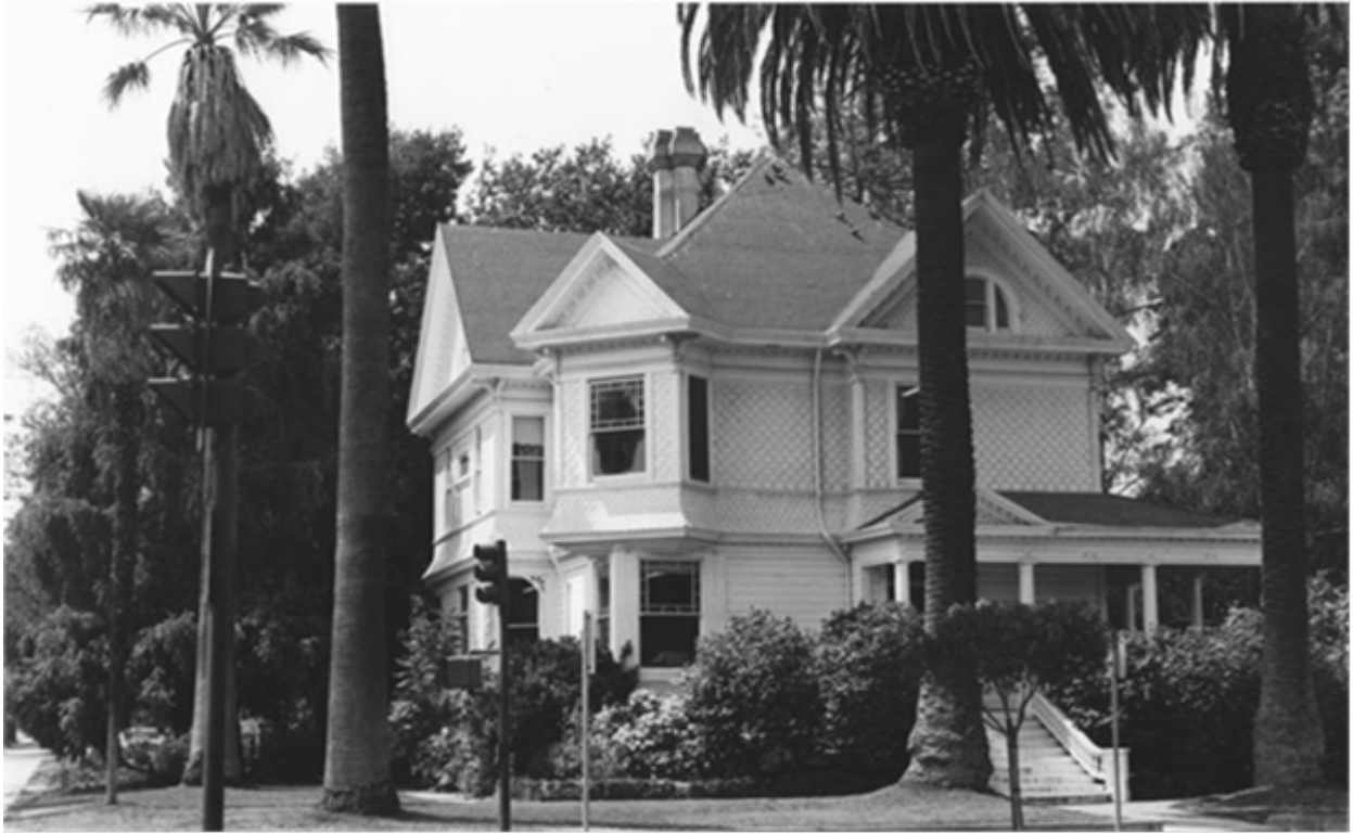
Figure 4 Recent York House Photo. Courtesy of Napa County Landmarks.
