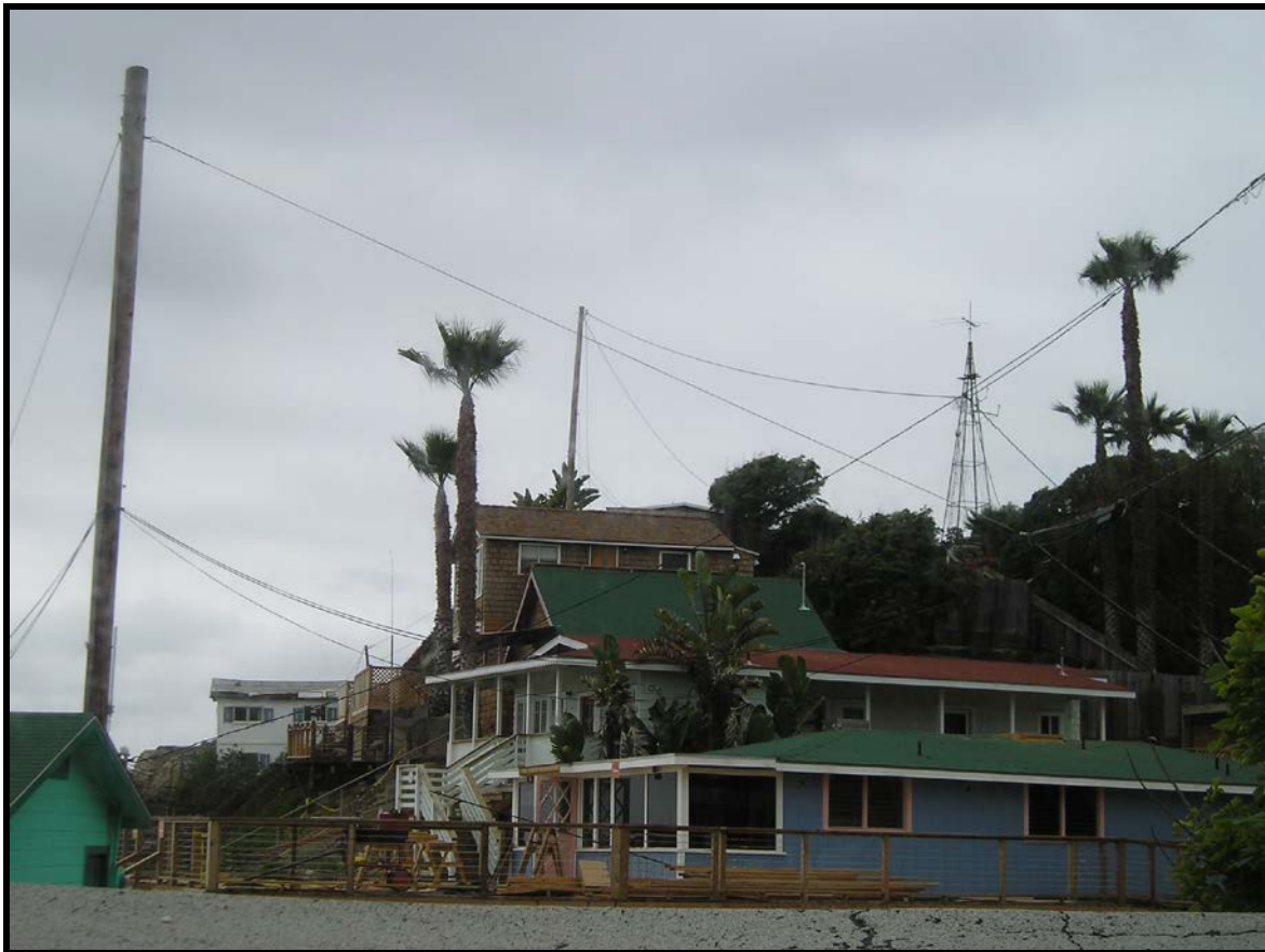
View north from Commons toward Cottages L to R #15, 2, 27, 24. Power poles, wires, and vegetation enhance the historic landscape, 2006.
