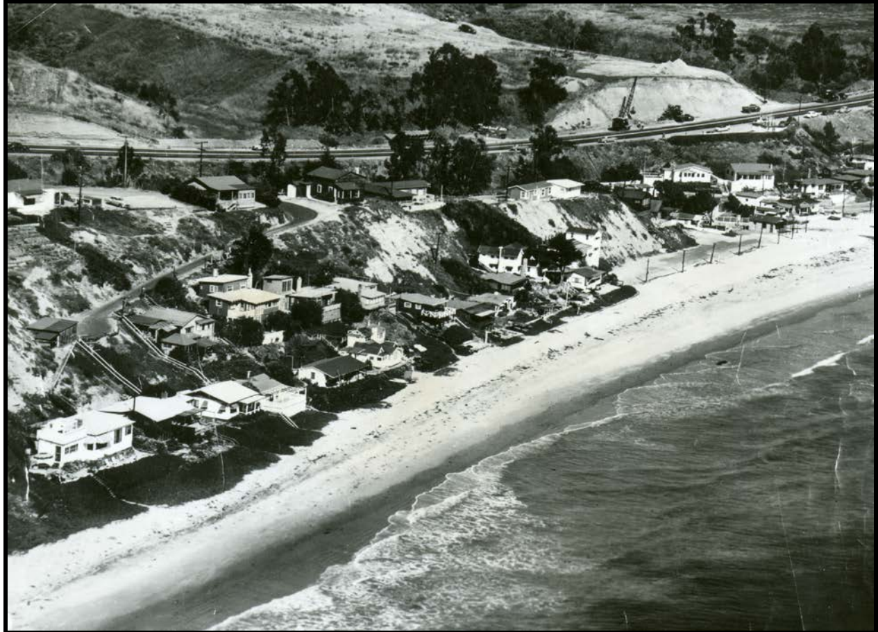
Aerial view southeast showing North Beach, Bluff-top, Beachfront, portion of South Beach, circa 1952.
