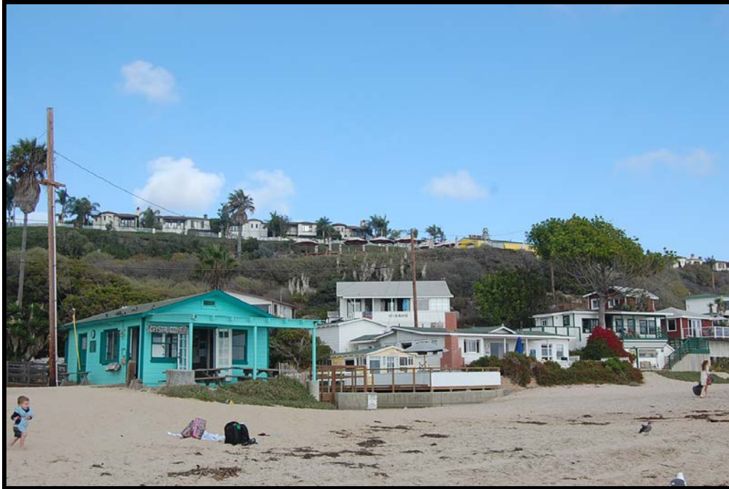
View southeast from beach toward South Beach, Cottages L to R #46, 40, 1, and 37; 19 and 16 above; 2013.
