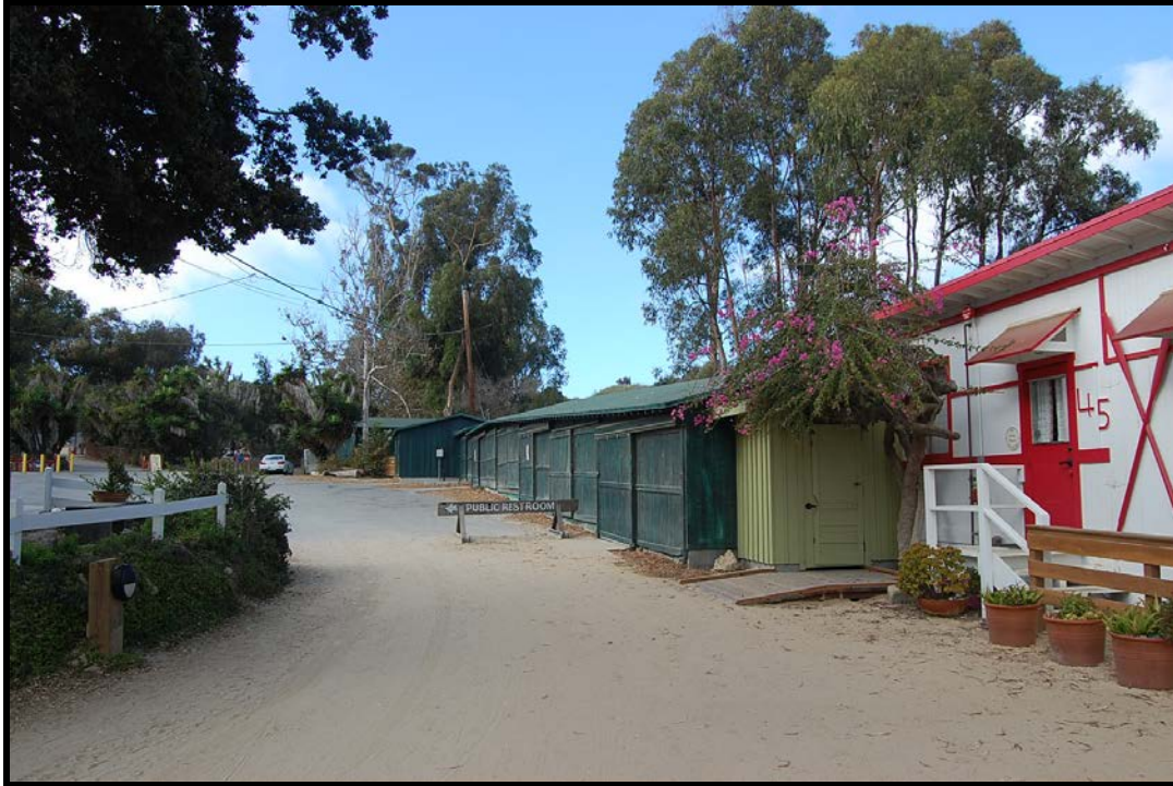
View east from between Cottages #5 and 45, toward Garages, 2013.
