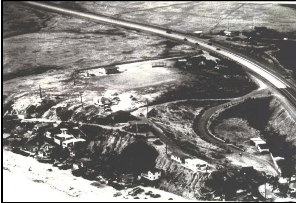
Aerial photo showing North Beach and Bluff-top late 1930s. Note Japanese Schoolhouse at upper center, not yet moved into district.
