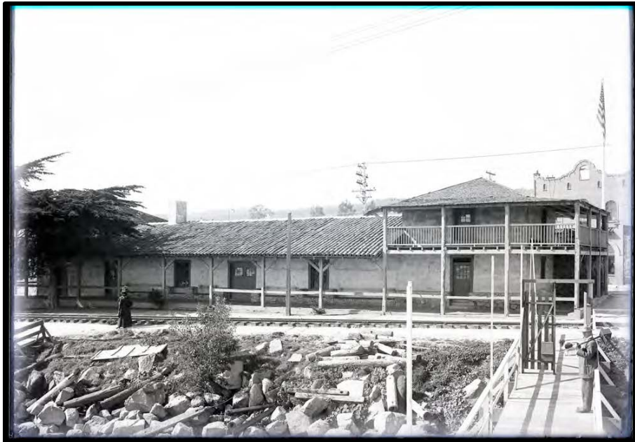
Custom House in 1909 showing completed repairs on the east side. Middle section roof is tile, while north and south ends remain wood shingle. Gift of Mary Holmgren, Monterey District, California State Parks, Monterey.
