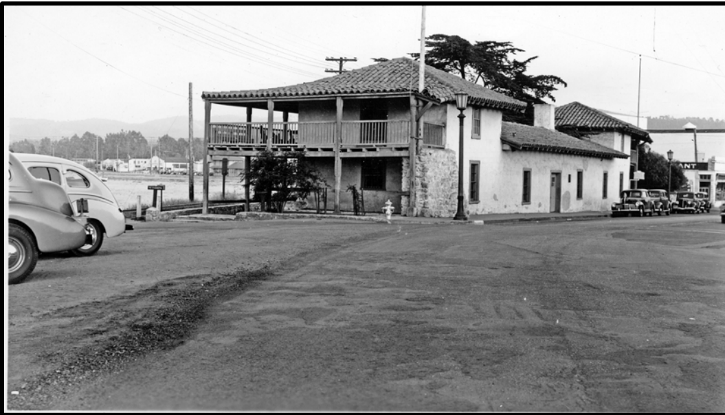
"Custom House, May 26, 1940. William L. Morgan, photographer. Morgan Collection. Photograph # MO-517-G. Courtesy California History Room Archives, Monterey Public Library. Note Alvarado Street on right and Fisherman's Wharf driveway north of the Custom House.
