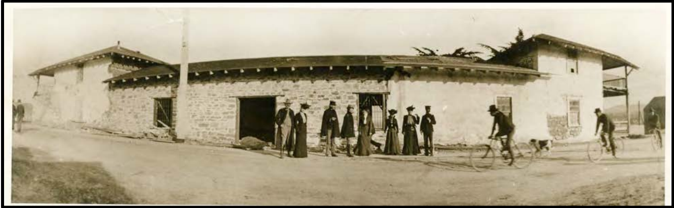
West side of Custom House in 1905 showing newly reconstructed middle section in stone. Note also that roof appears to be in process of being replaced. Monterey District, California State Parks, Monterey.
