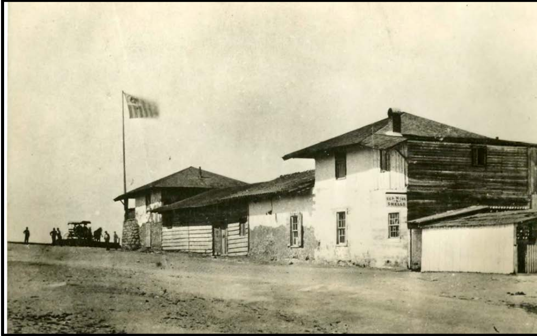
Oldest known photograph of the Custom House showing the west side, undated, believed to be circa 1867. A Customs Service flag appears to be flying at the flagpole on the northwest corner. Weatherboard siding installed in the 1850s is evident. Southern end has been boarded up to provide additional living space for the caretaker. Note also shingle roofs except for southern portion of central section. Monterey District, California State Parks, Monterey.
