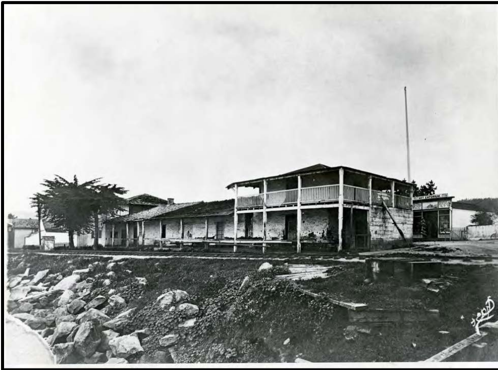
East side of the Custom House following the construction of the railroad, circa 1890s. Monterey District, California State Parks, Monterey
