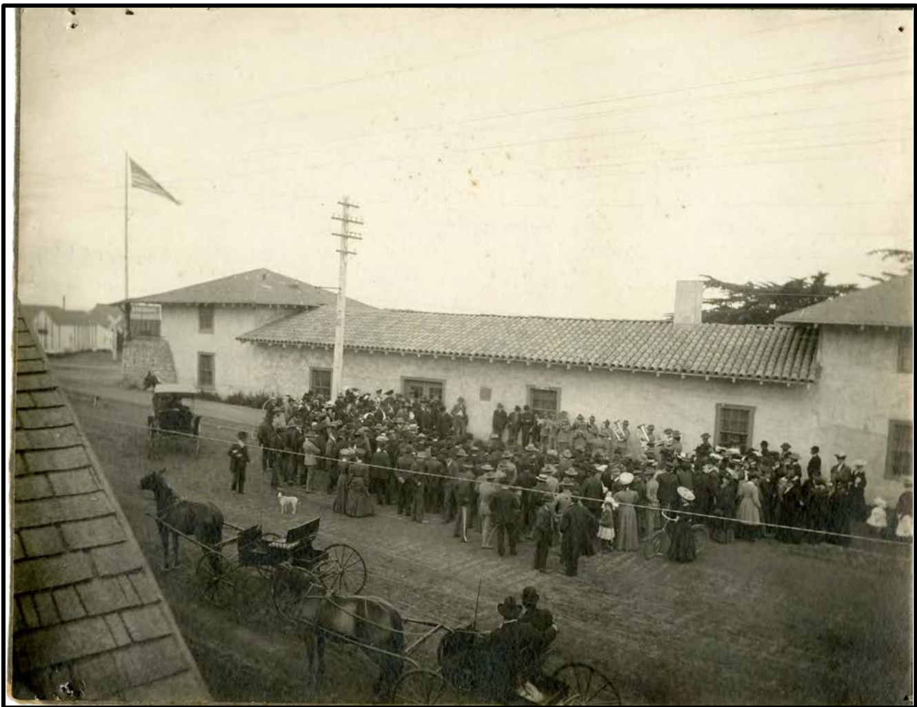
West side of Custom House for plaque dedication, 1905. Note tile roof in middle section is complete, as are new windows and doors on this same section. Monterey District, California State Parks, Monterey.
