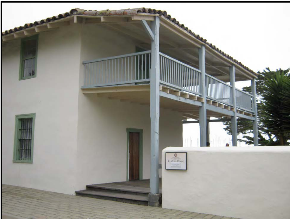
South elevation. Photograph by Garavaglia Architecture, Inc., May 2010 for Monterey Custom House Historic Structure Report .
