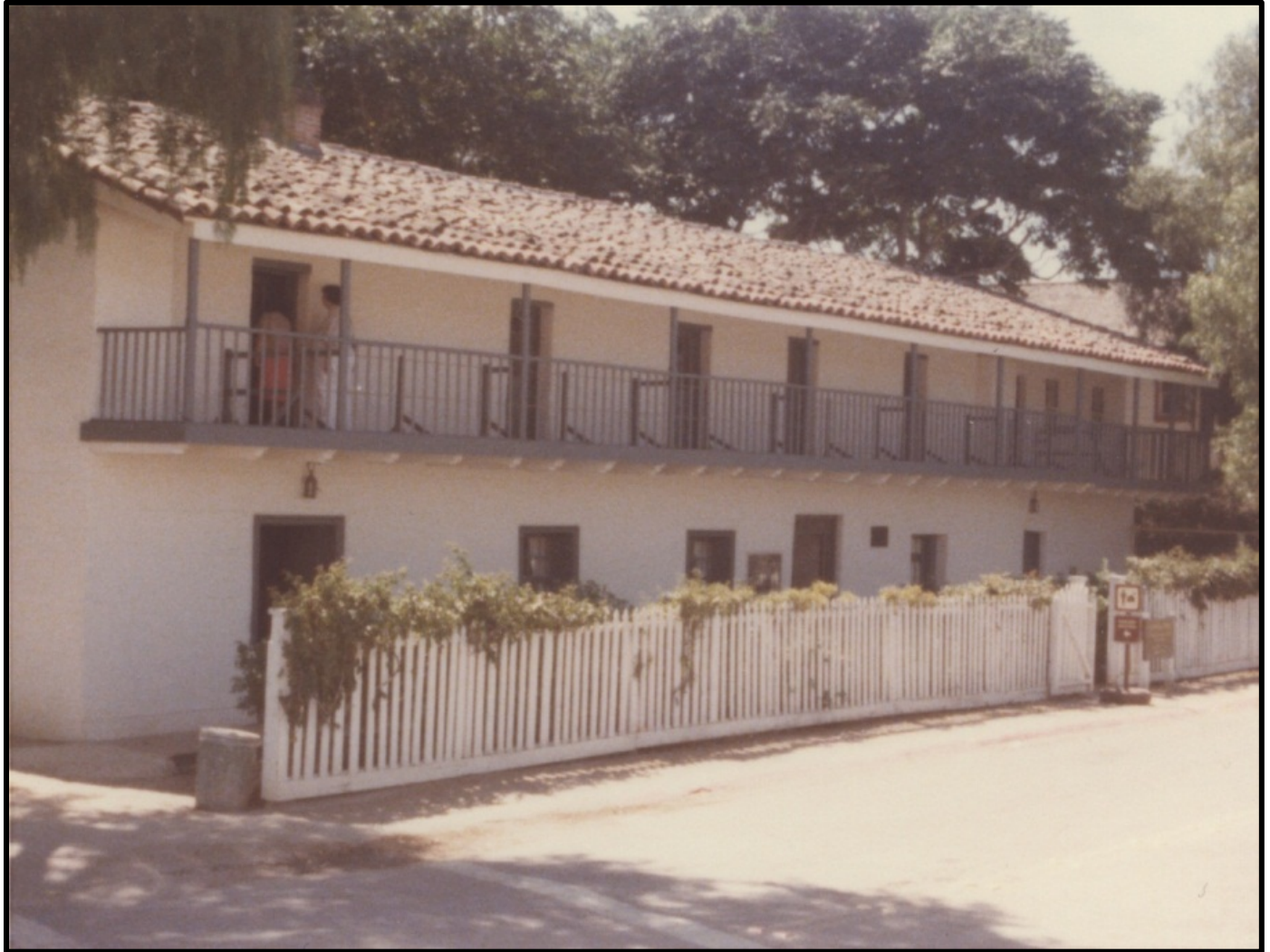
Castro-Breen Adobe, north elevation, San Juan Bautista Historic Park, 1979. Source: CHL #0179 nomination file.
