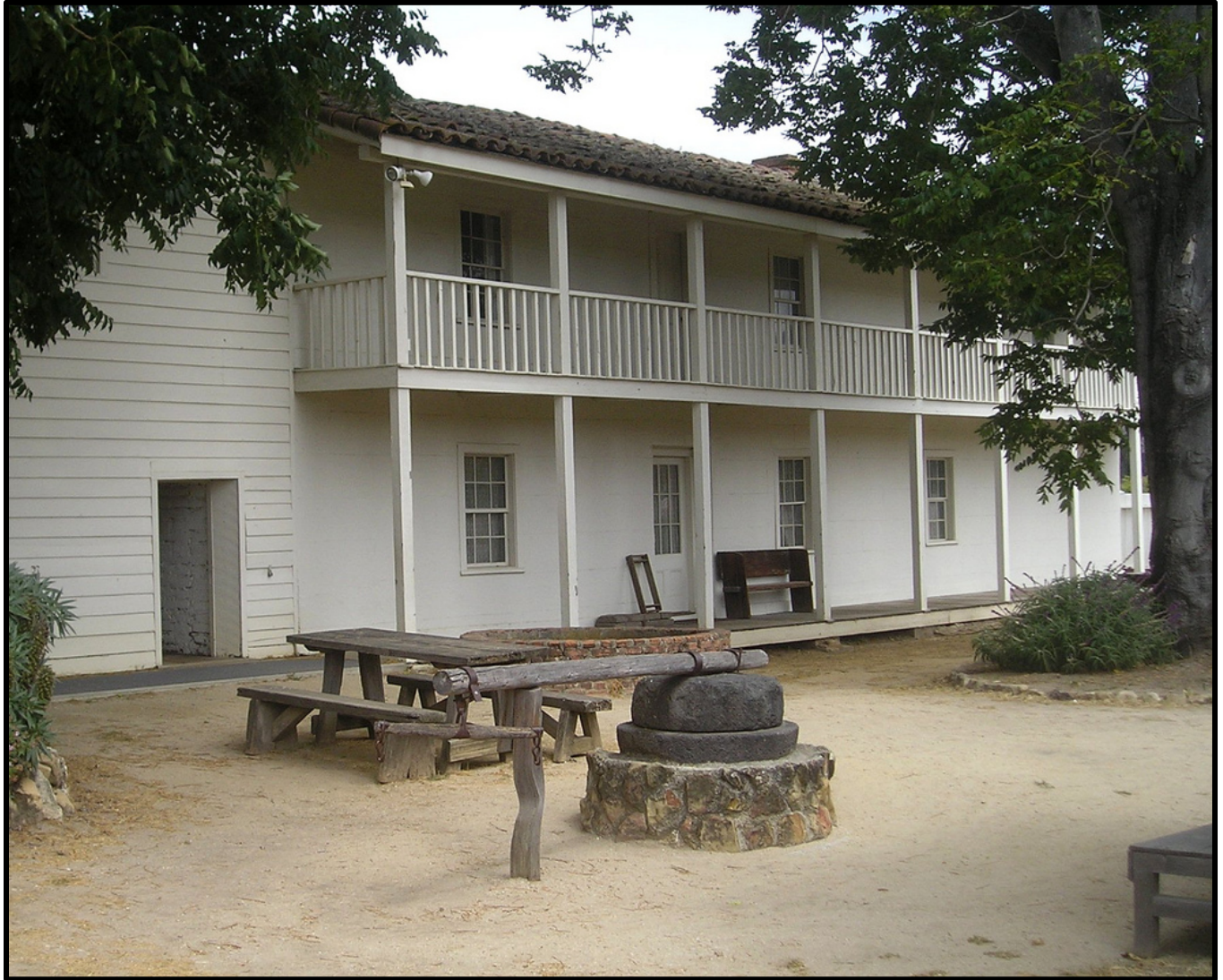
Castro-Breen Adobe, south elevation, San Juan Bautista Historic Park, post-rehabilitation, circa 2003.
