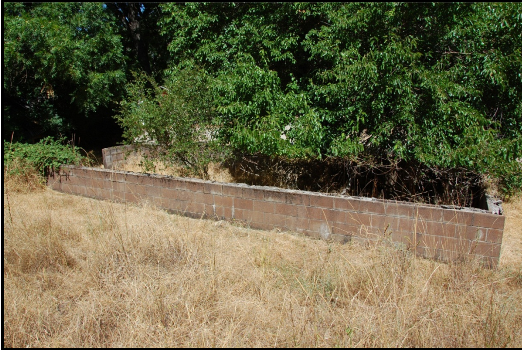
Photo 10. Foundation remains of the Harrison greenhouse. Photographed by David Anderson, June 2012.
