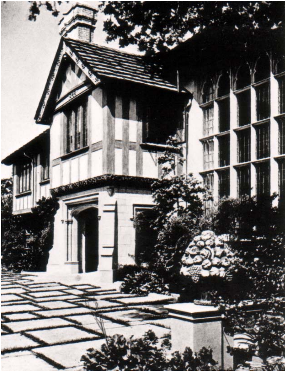
Detail of main entry (north façade), 1931. Source: California Arts and Architecture
