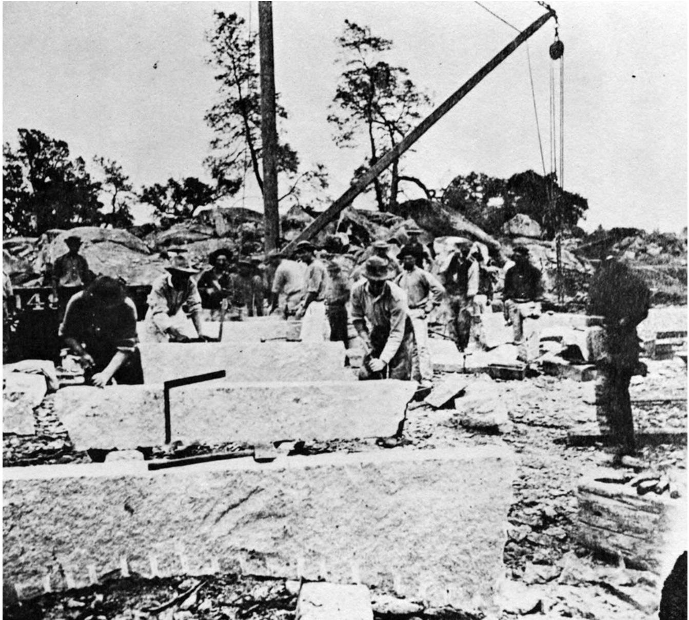
Figure 3: Historic photograph (ca 1900) depicting granite workers chiseling granite slabs beside granite quarry with derrick and rail car in background.
