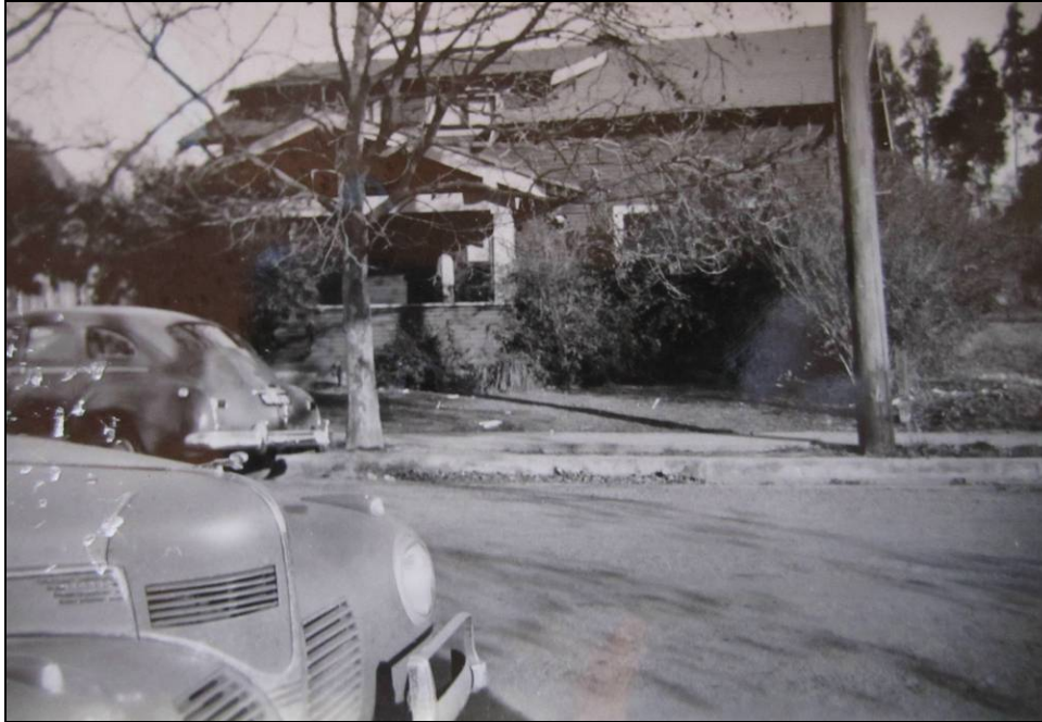
Figure 21. Photographs of west (front) and south façades, circa 1940
