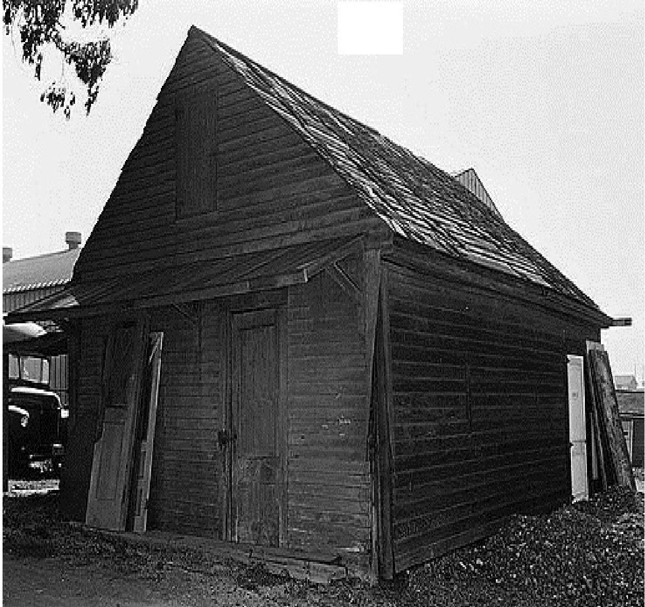
Figure 3. View south of southern and eastern façades; photographer and date unknown. Courtesy City of Benicia.
