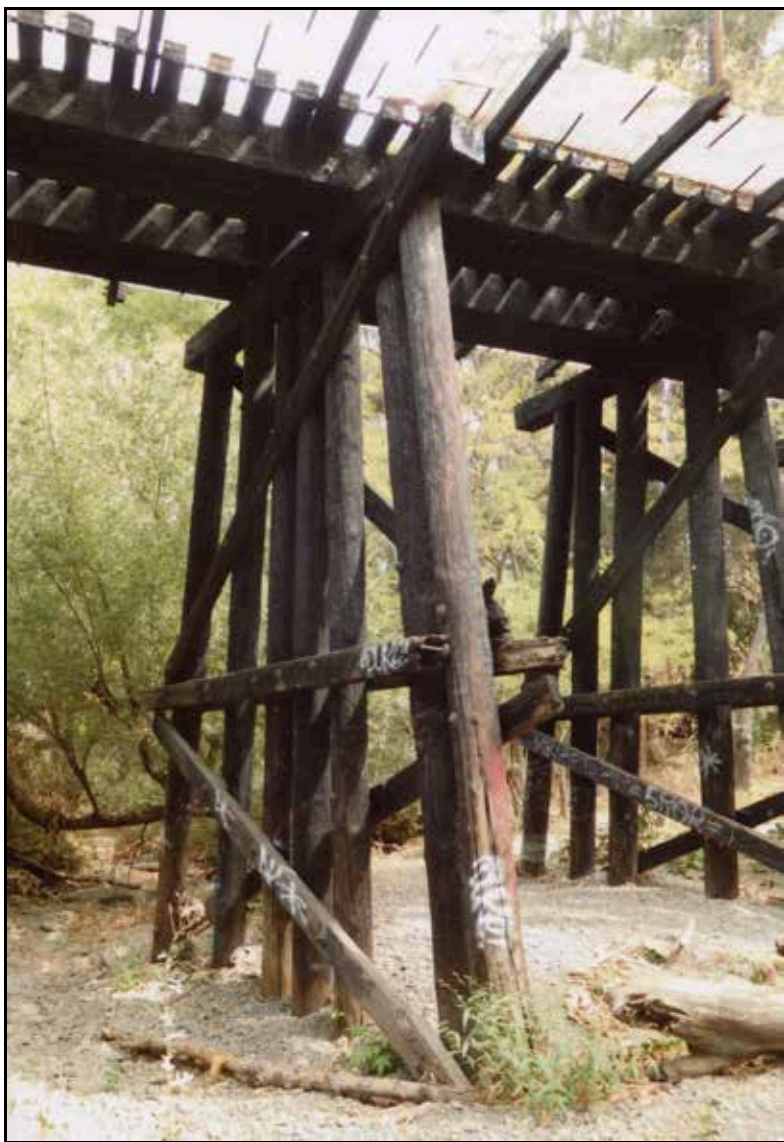
Figure 11. View of Willow Glen Trestle, Bent 8, looking east.
