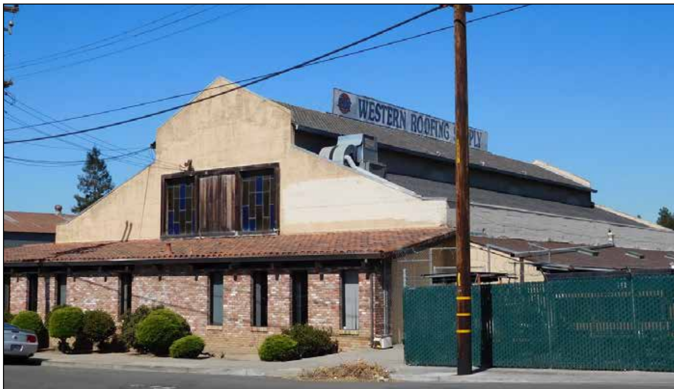
Figure 8. Hamlin Packing Company building located at 991 Lonus Street as it appears today.
