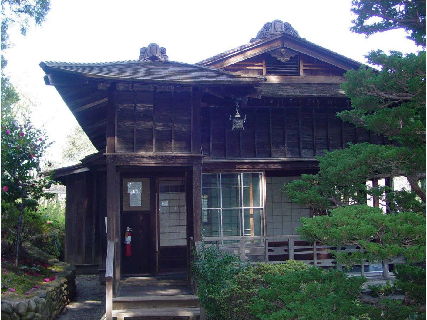
Spring View northeast at Upper House.
