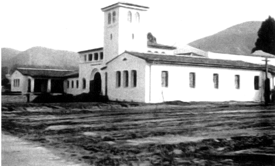
Figure 2: 1936 Photograph of completed building
