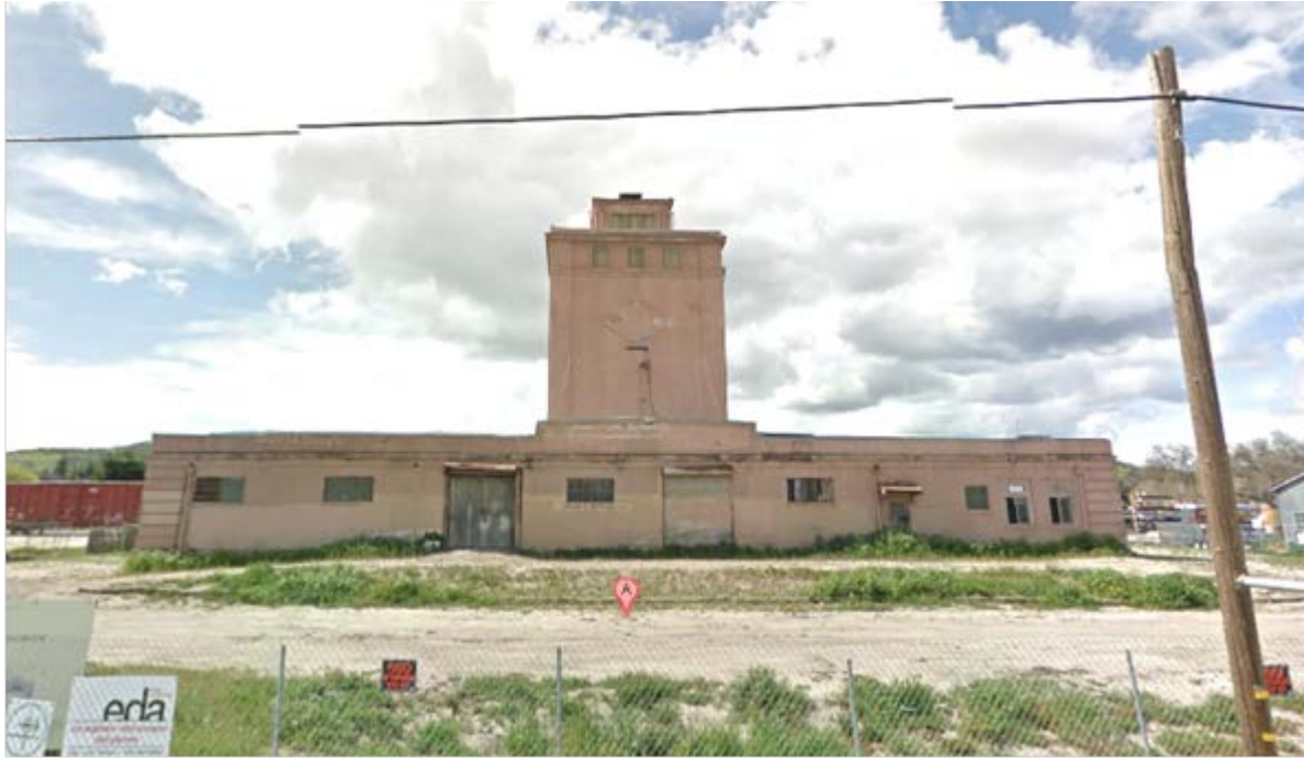
Figure 11. East elevation, view to the west. (Google, March 2012)
