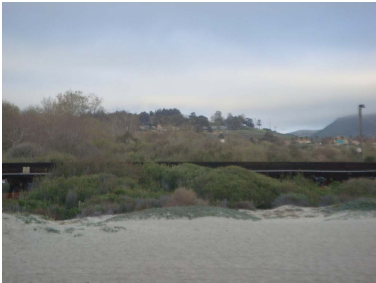
CA_San Diego County_Trestles Historic District_0035 Upper Trestles, northern Atchison, Topeka & Santa Fe Railroad trestle, looking northwest
