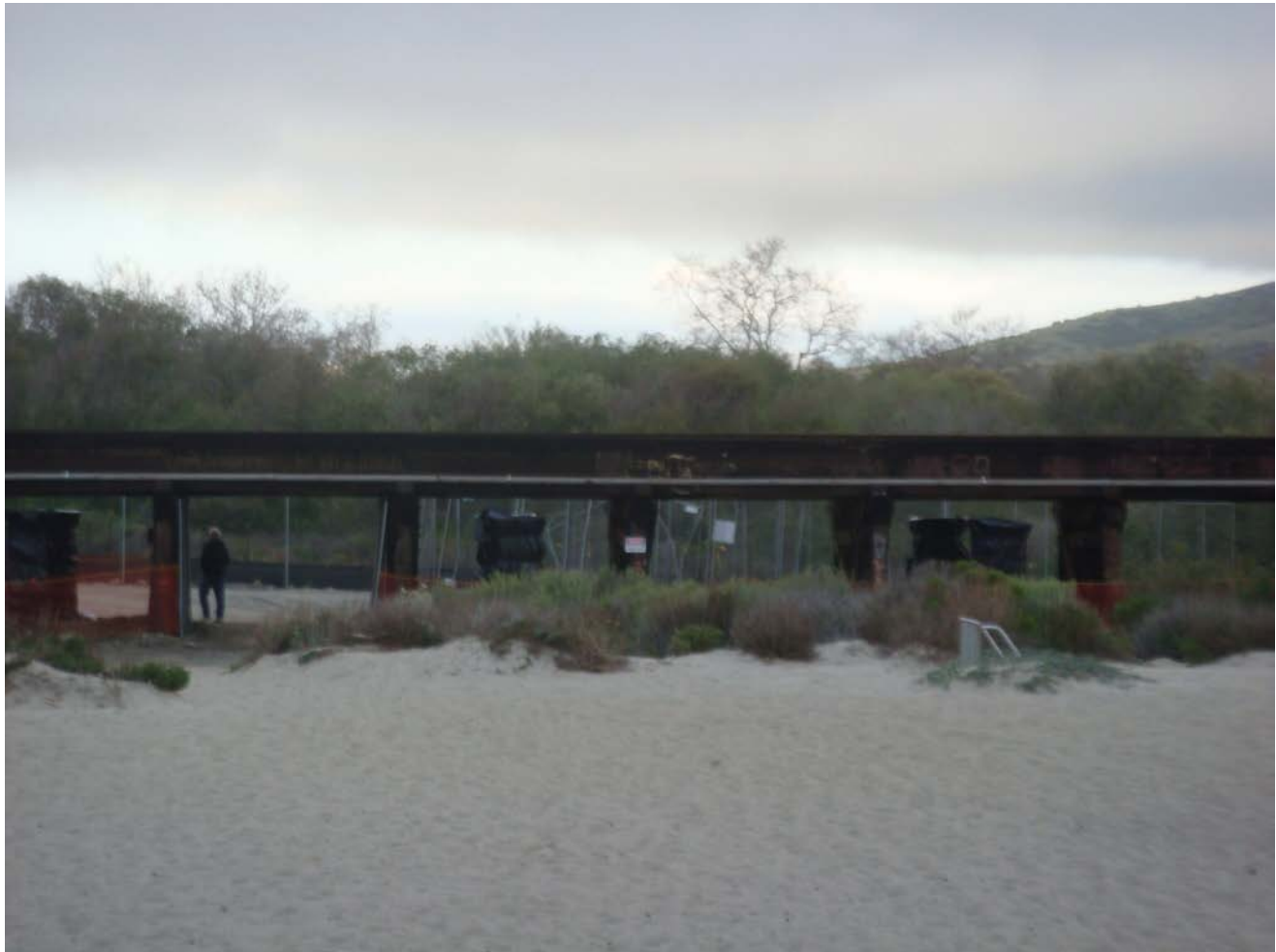
CA_San Diego County_Trestles Historic District_0037 Upper Trestles, northern Atchison, Topeka & Santa Fe Railroad trestle, looking north
