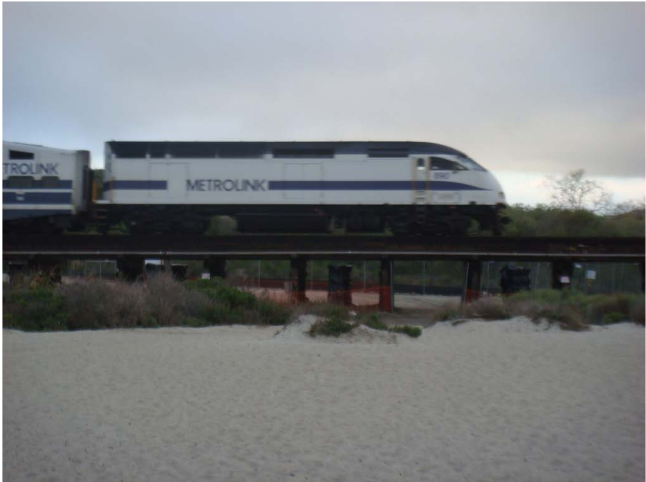
CA_San Diego County_Trestles Historic District_0039 Metrolink train on Atchison, Topeka & Santa Fe Railroad trestle, looking northeast
