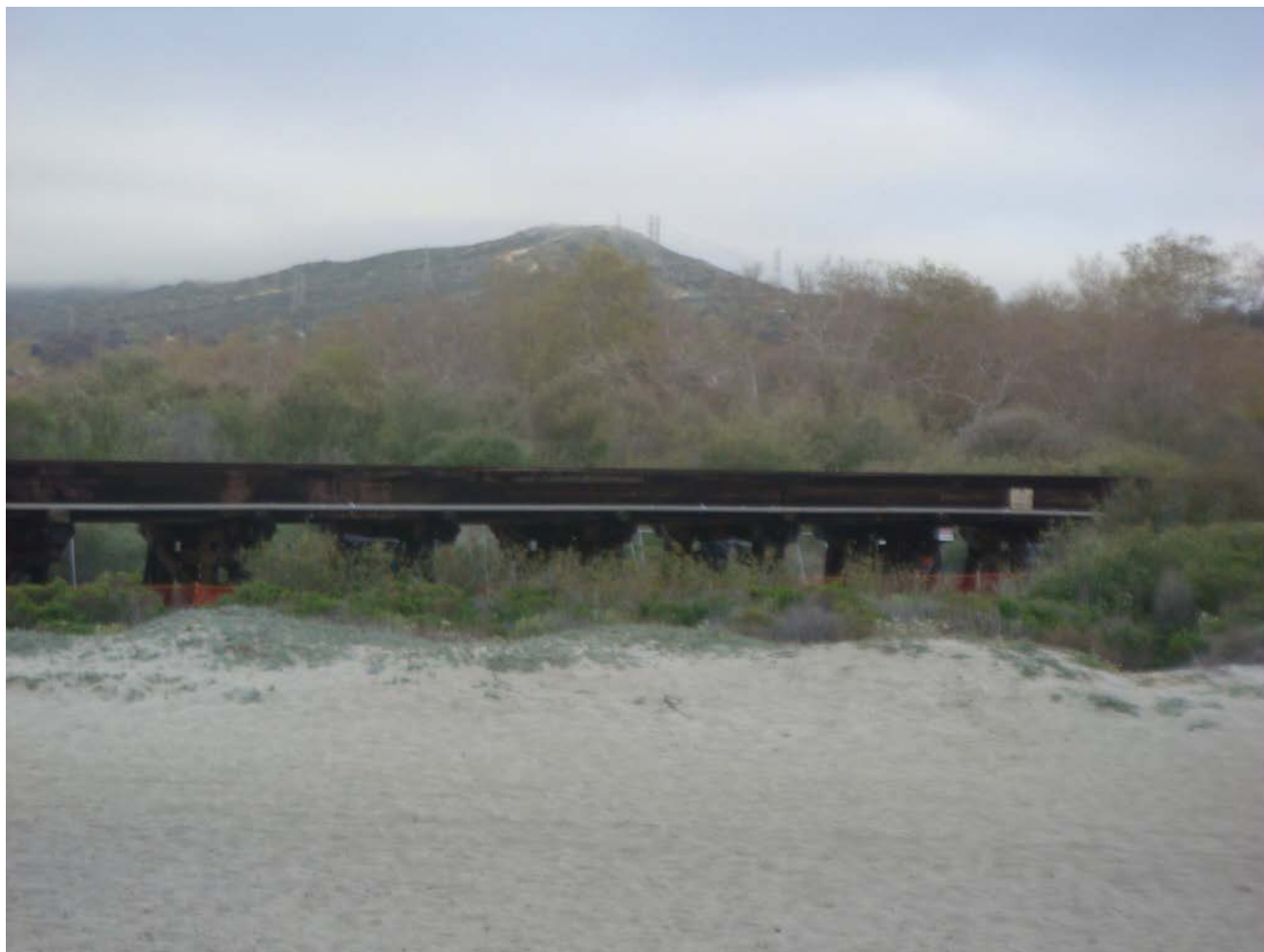
CA_San Diego County_Trestles Historic District_0036 Upper Trestles, northern Atchison, Topeka & Santa Fe Railroad trestle, looking northwest
