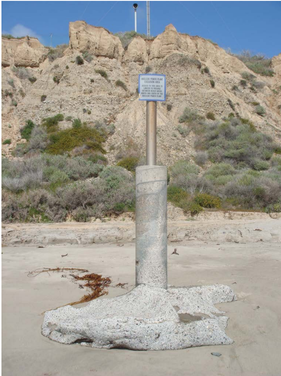
CA_San Diego County_Trestles Historic District_0026 Southernmost corner of nominated district, looking northeast
