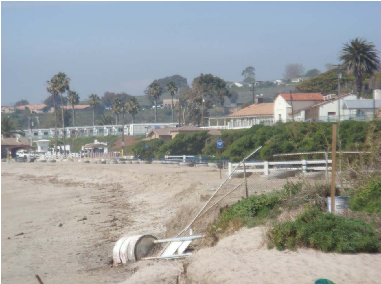
CA_San Diego County_Trestles Historic District_0013 Church, U.S. Marine Corps (USMC) facilities, looking north
