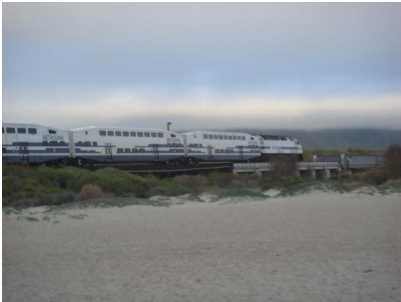
CA_San Diego County_Trestles Historic District_0040 Metrolink train on Atchison, Topeka & Santa Fe Railroad trestle, looking east
