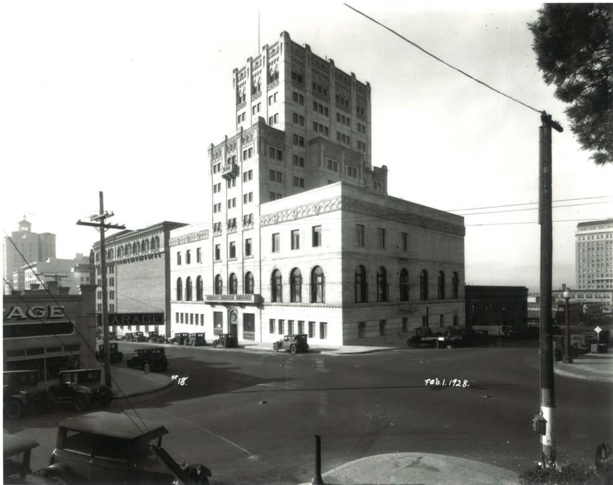
San Diego Athletic Club 1250 Sixth Avenue, San Diego County CA 1928 Photograph of East and North Facades
