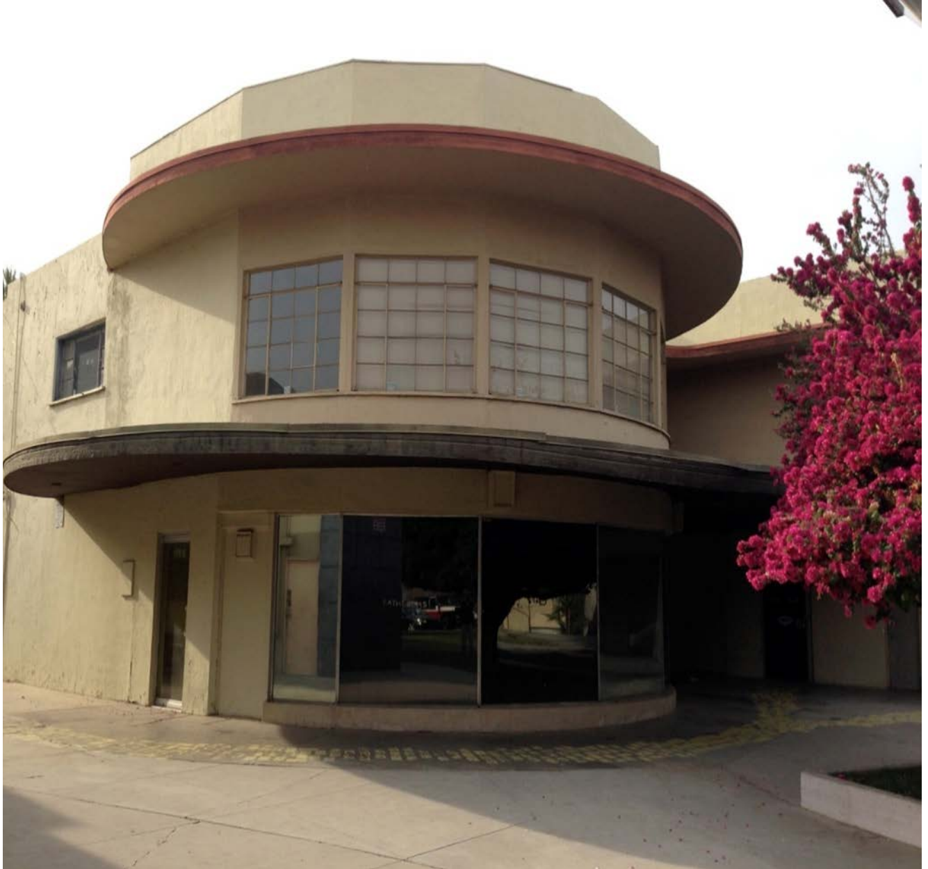
Photo 9. In the courtyard looking northwest toward Building A (Twin Building North), May 2014
