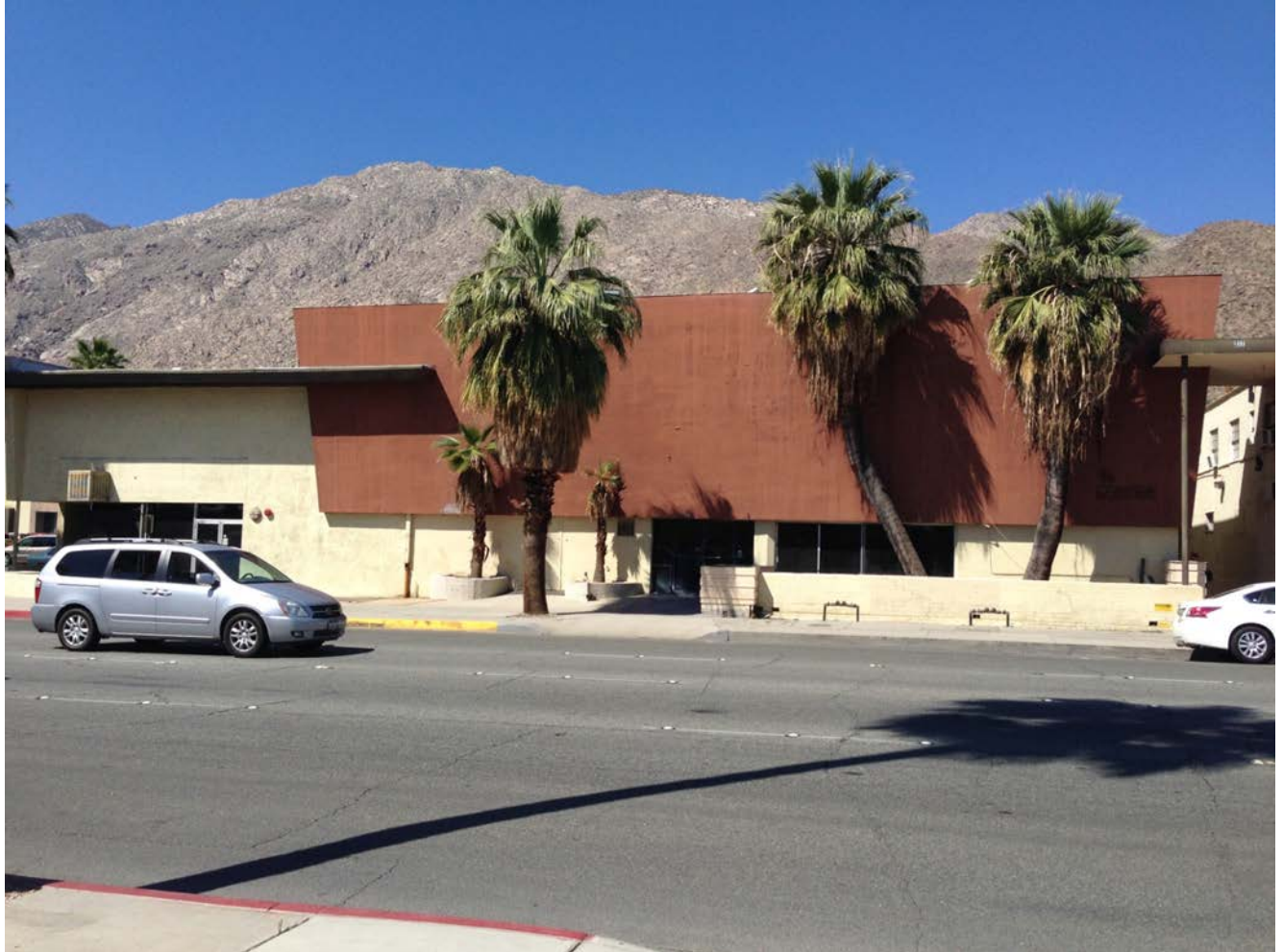
Photo 4. Indian Canyon Drive, looking west towards Building D (with a portion of Building A to the north), May 2014
