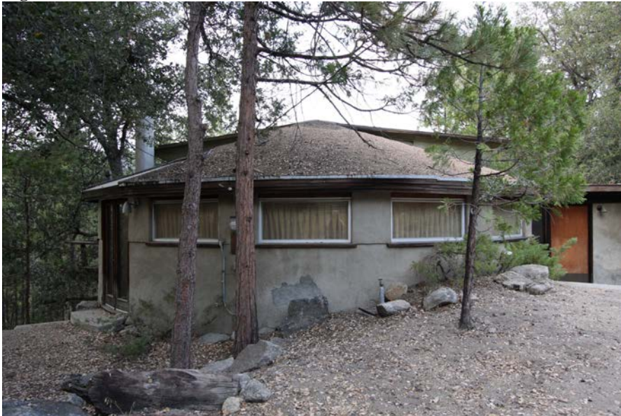
View of south façade, facing north (Photo credit: Flickr – James, photographed in 2008)
