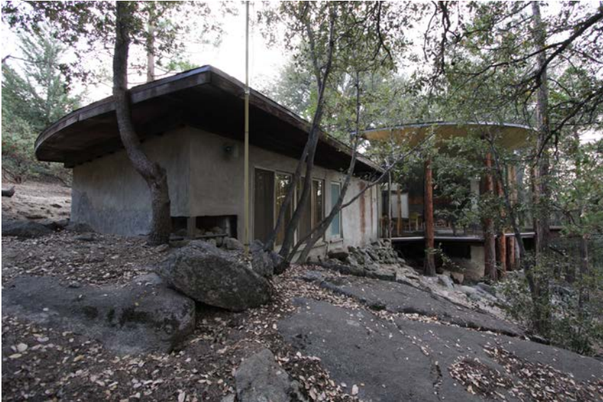
View of west and north façade, facing west (Photo credit: Flickr – James, photographed in 2008)
