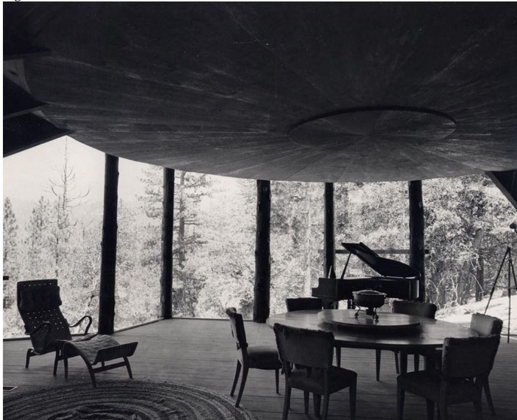
Interior detail of living room and sawtooth windows (© The John Lautner Foundation, courtesy of Frank Escher, date of photograph unknown)
