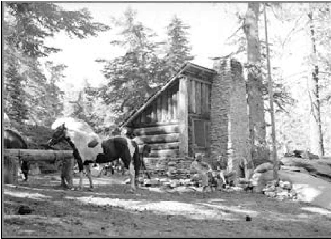
Photograph # HP11 Looking North at Round Valley Shelter Date: 1952 August Source: CA State Museum Accession # 090-23420
